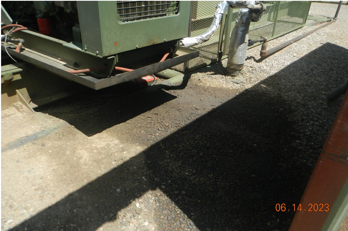
Photo 3. Stained soils were also observed near the engine compressor where the leak appeared to have come from.
