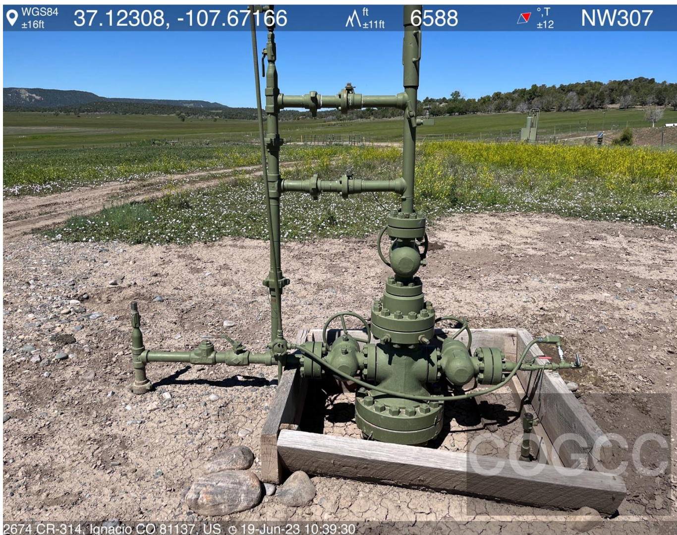
Photo #2 View of the wellhead assembly.
