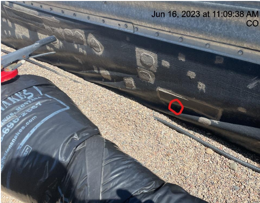
Photo # 835 Hole in containment line/liner needs maintenance
