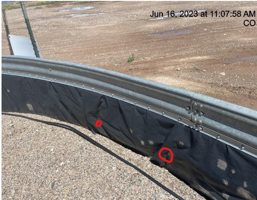
Photo # 829 Holes in containment line/liner needs maintenance
