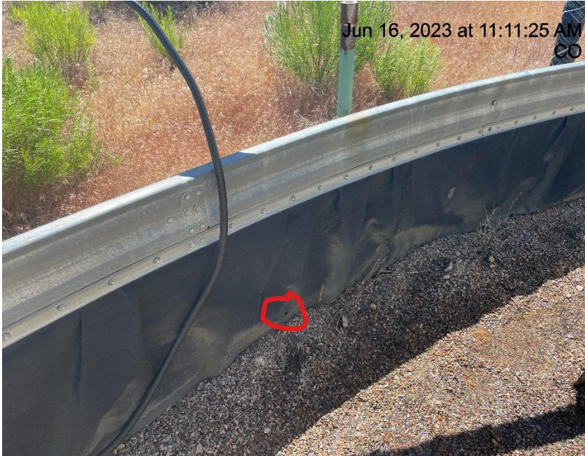
Photo # 847 Hole in containment line/liner needs maintenance
