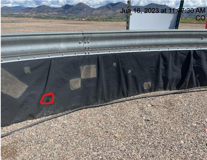
Photo # 825 Hole in containment line/liner needs maintenance
