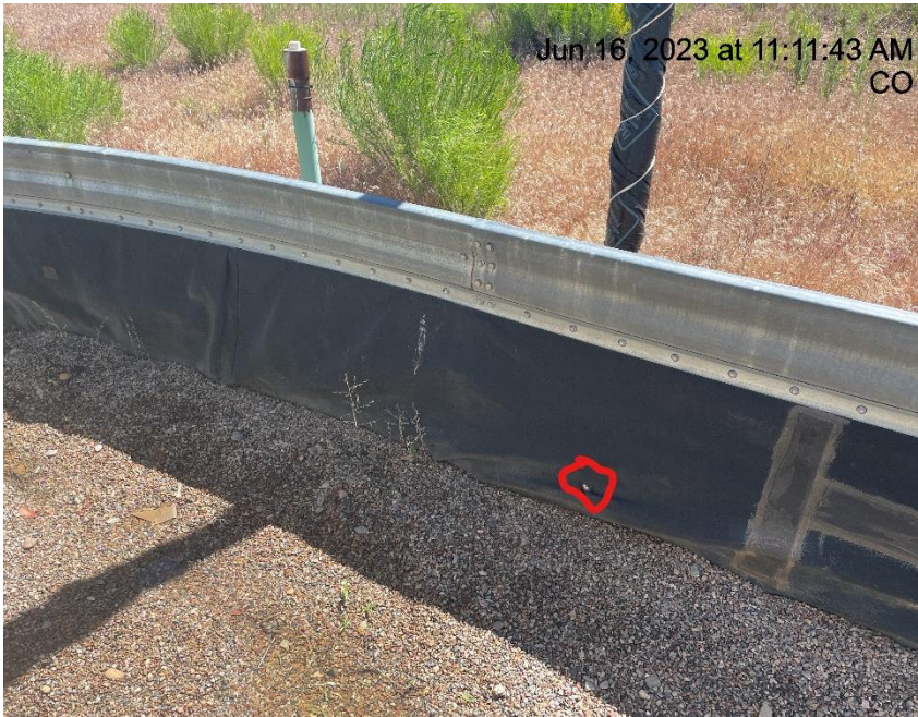
Photo # 849 Hole in containment line/liner needs maintenance
