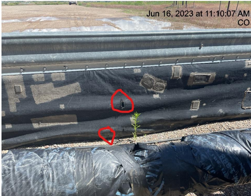
Photo # 837 Holes in containment line/liner needs maintenance
