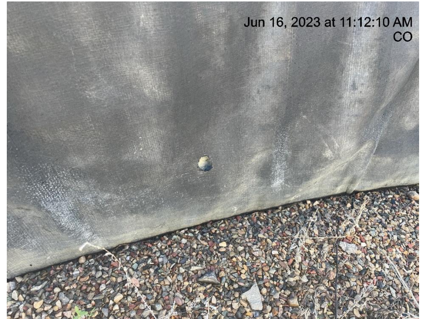
Photo # 854 Hole in containment line/liner needs maintenance
