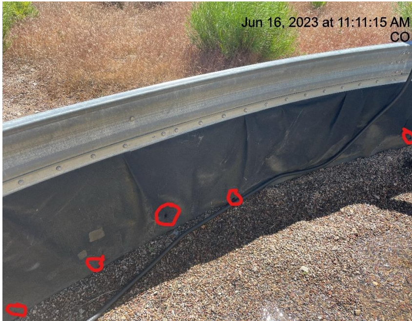
Photo # 845 Holes in containment line/liner needs maintenance
