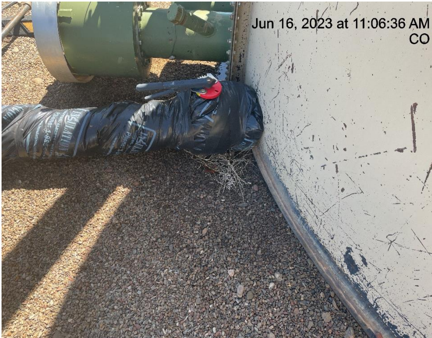
Photo # 823 Stained gravel in secondary containment
