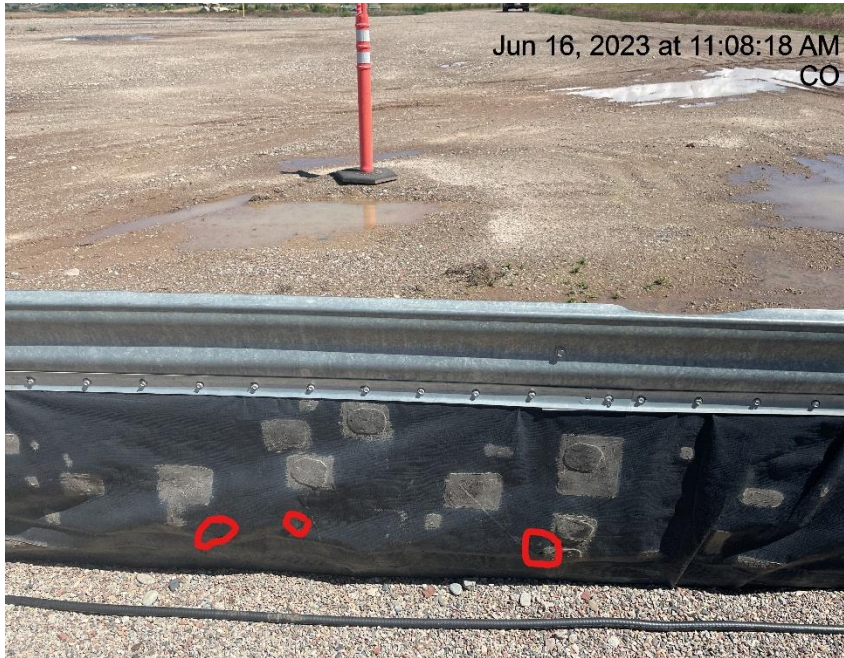
Photo # 832 Holes in containment line/liner needs maintenance
