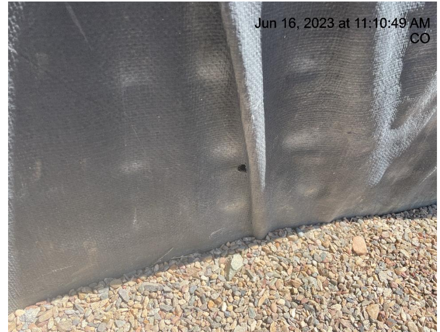
Photo # 842 Hole in containment line/liner needs maintenance
