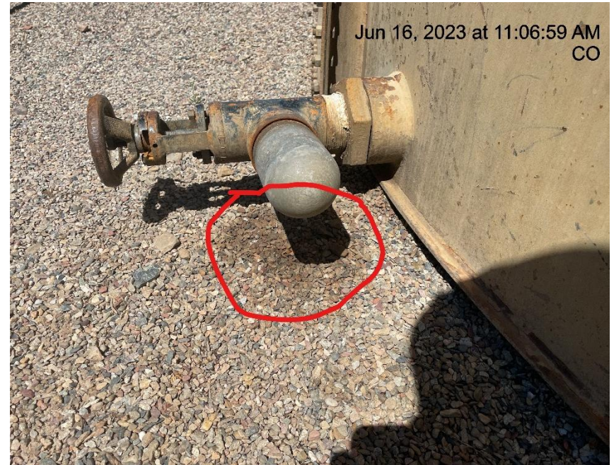
Photo # 824 Stained gravel in secondary containment
