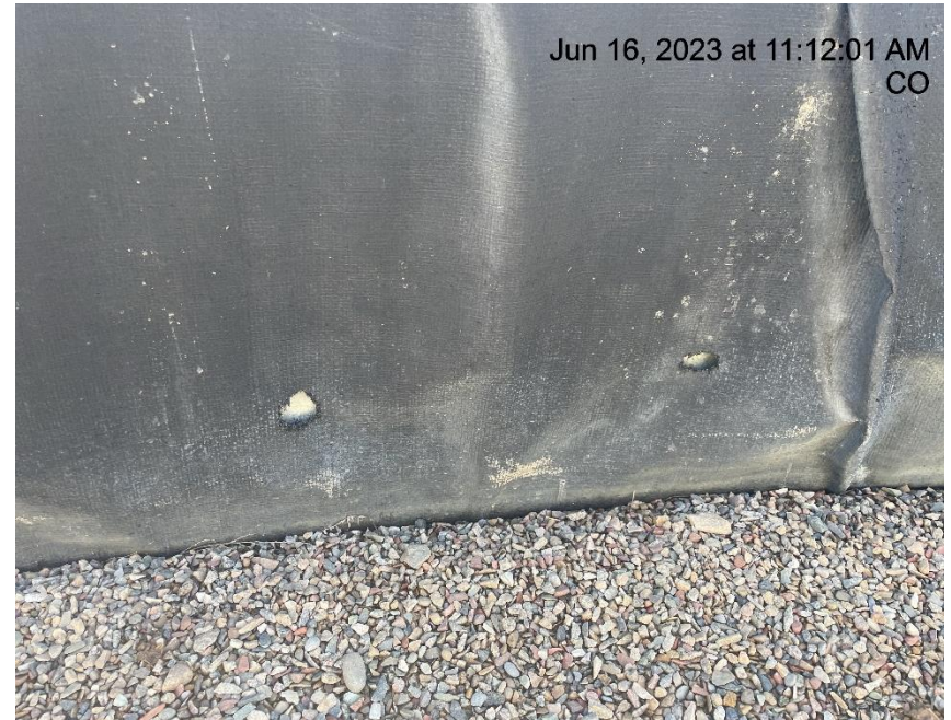
Photo # 852 Holes in containment line/liner needs maintenance
