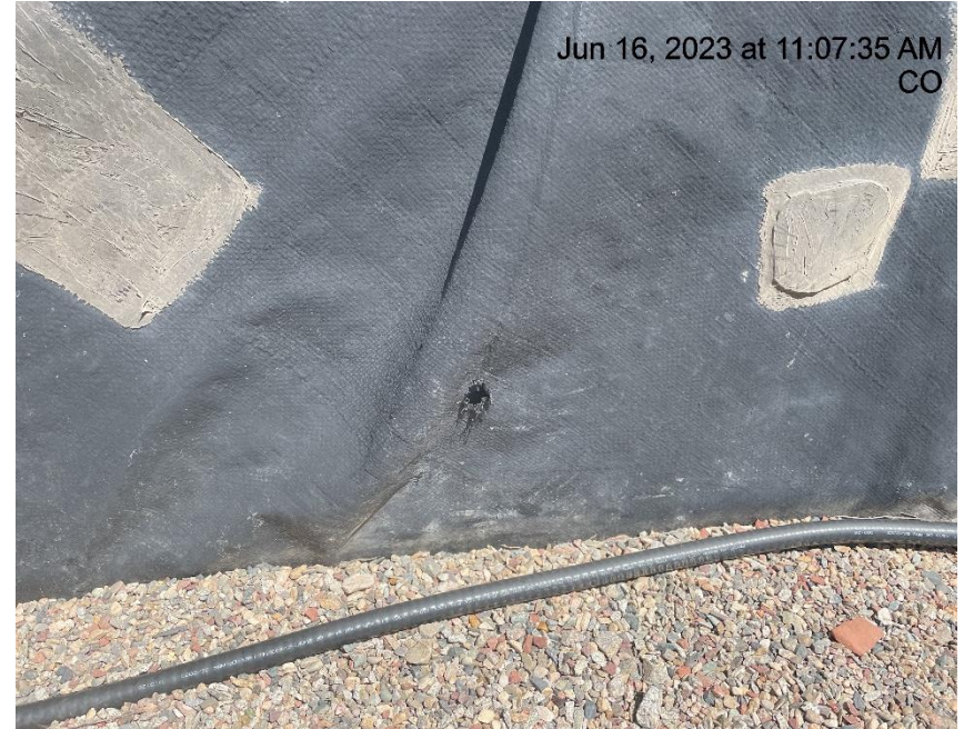
Photo # 826 Hole in containment line/liner needs maintenance
