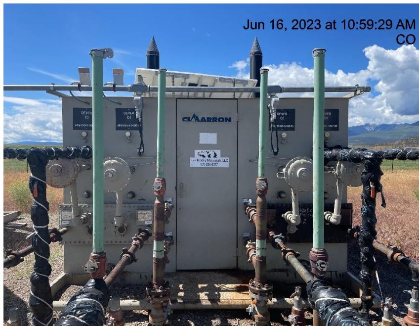
Photo # 799 Meter calibration info not conspicuously posted
