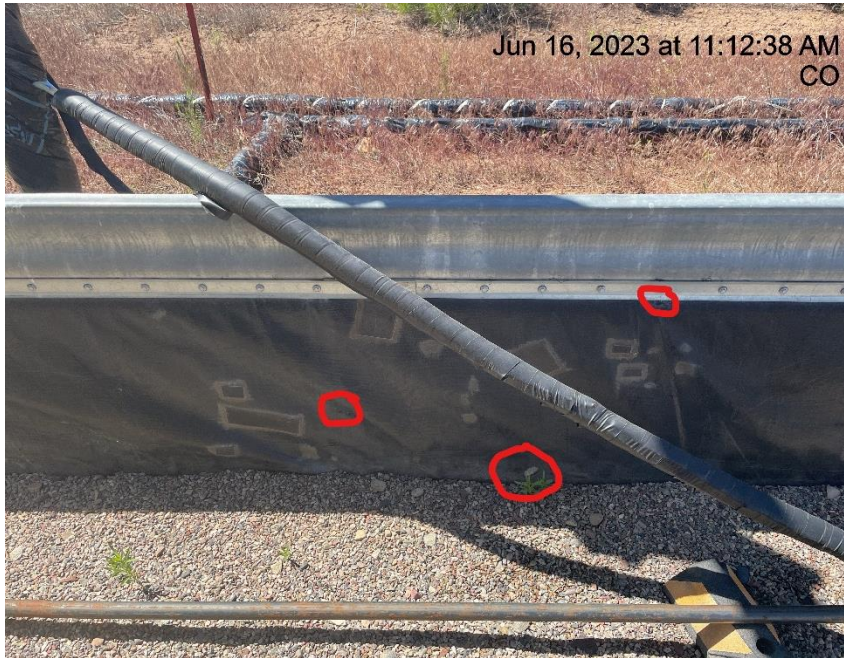
Photo # 855 Holes in containment line/liner needs maintenance
