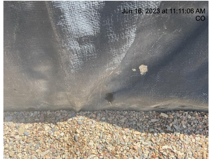
Photo # 844 Hole in containment line/liner needs maintenance
