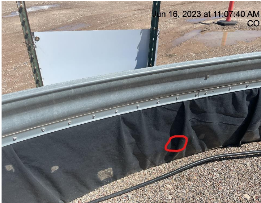
Photo # 827 Hole in containment line/liner needs maintenance
