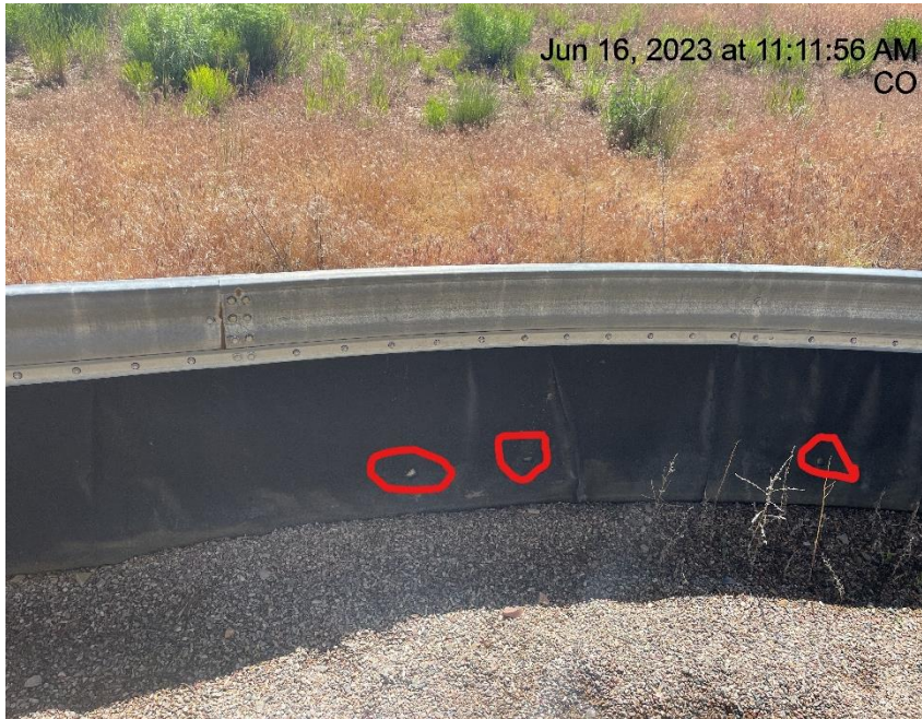
Photo # 851 Holes in containment line/liner needs maintenance
