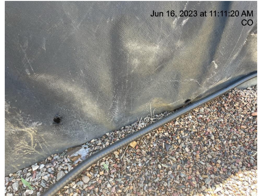
Photo # 846 Holes in containment line/liner needs maintenance
