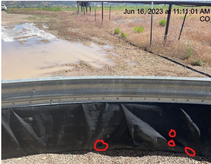
Photo # 843 Holes in containment line/liner needs maintenance
