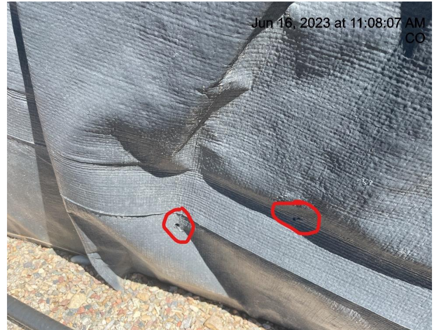
Photo # 831 Holes in containment line/liner needs maintenance
