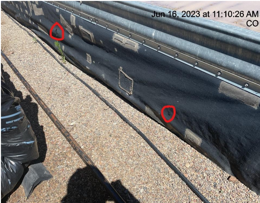
Photo # 839 Holes in containment line/liner needs maintenance
