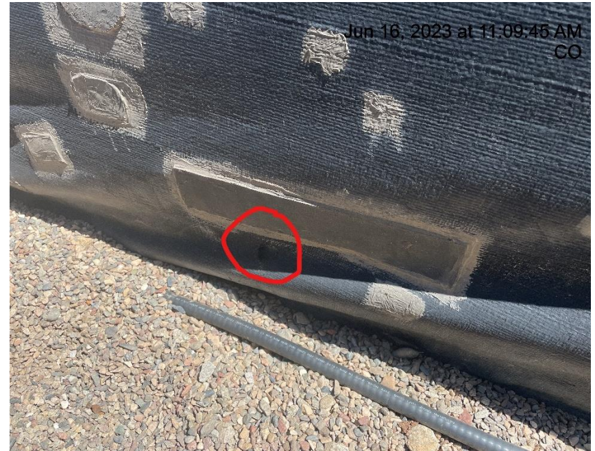
Photo # 836 Hole in containment line/liner needs maintenance
