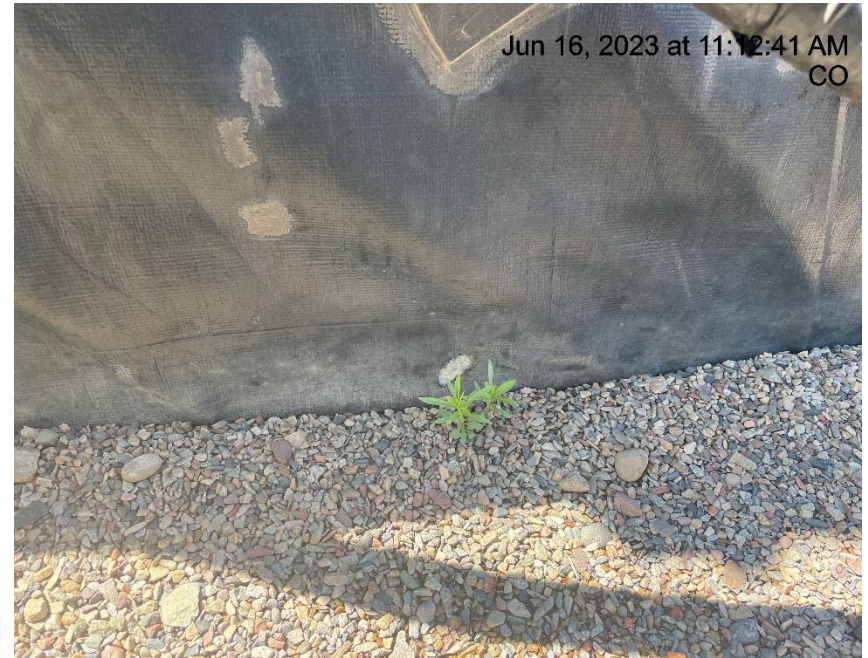
Photo # 856 Hole in containment line/liner needs maintenance
