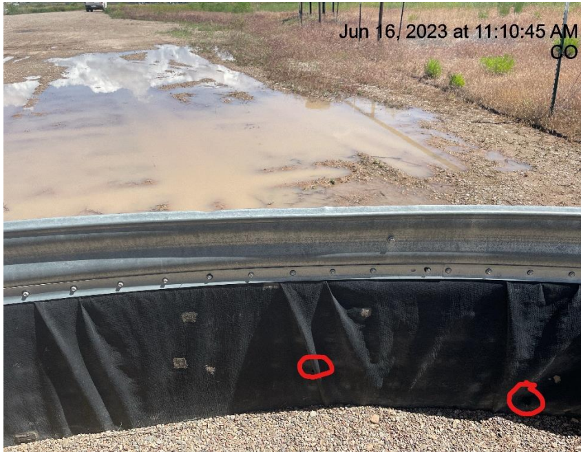
Photo # 841 Holes in containment line/liner needs maintenance
