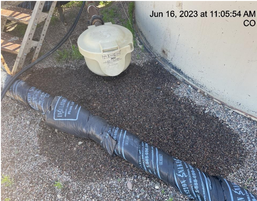
Photo # 818 Stained gravel in secondary containment
