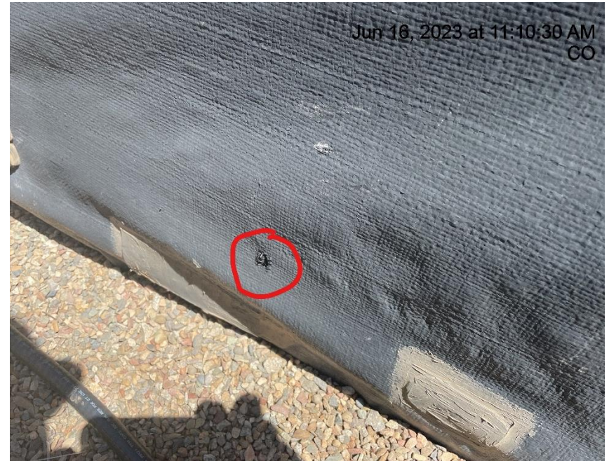
Photo # 840 Hole in containment line/liner needs maintenance
