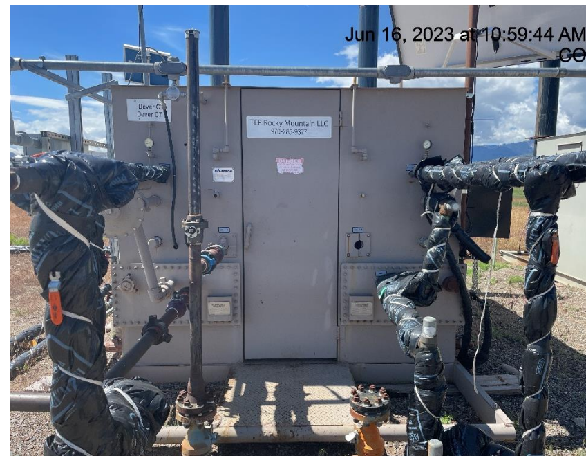
Photo # 800 Meter calibration info not conspicuously posted
