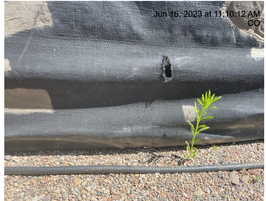
Photo # 838 Holes in containment line/liner needs maintenance
