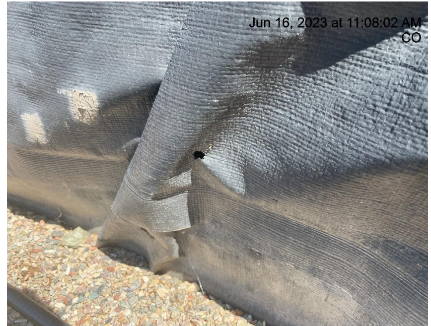
Photo # 830 Hole in containment line/liner needs maintenance
