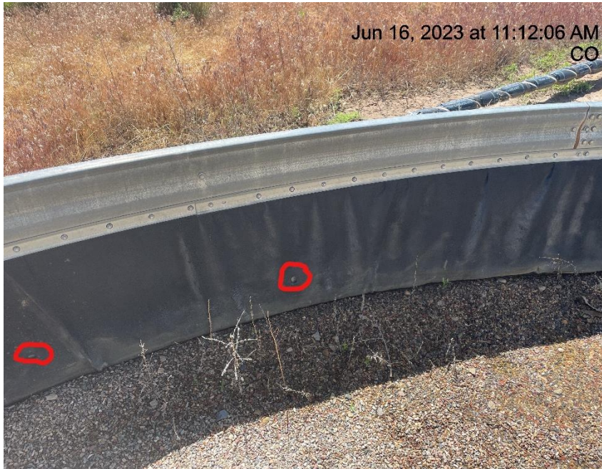
Photo # 853 Holes in containment line/liner needs maintenance
