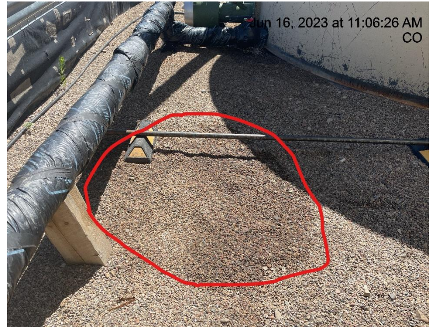
Photo # 821 Stained gravel in secondary containment
