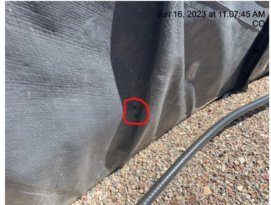
Photo # 828 Hole in containment line/liner needs maintenance
