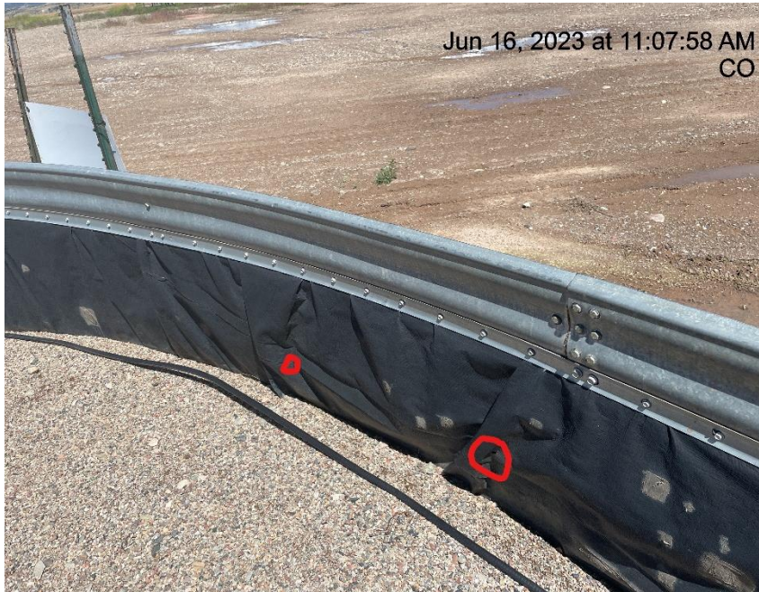
Photo # 829 Holes in containment line/liner needs maintenance
