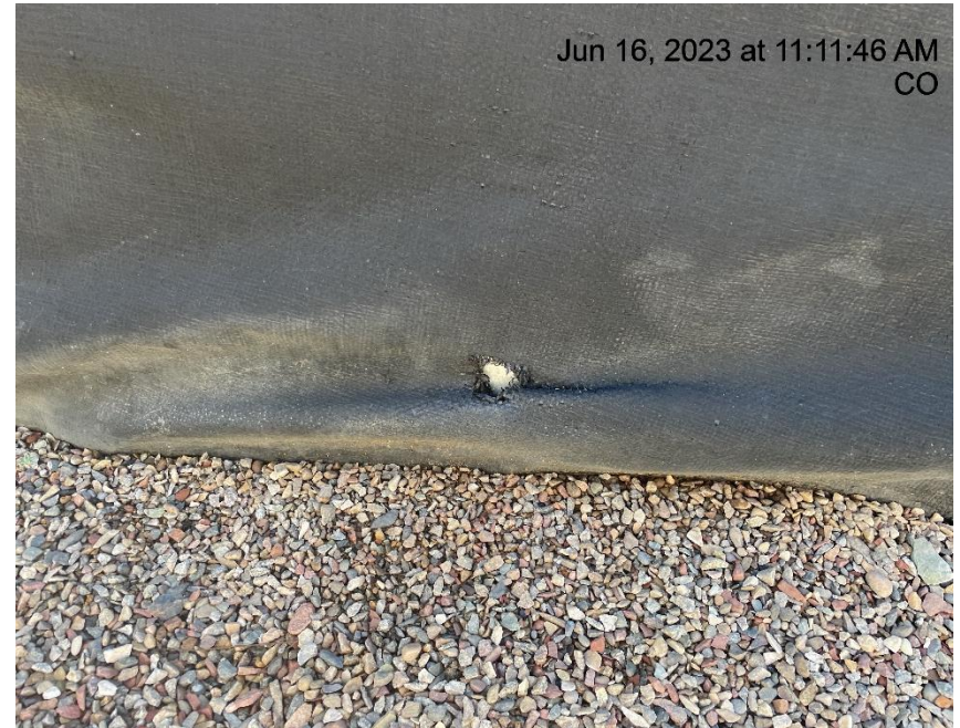
Photo # 850 Hole in containment line/liner needs maintenance
