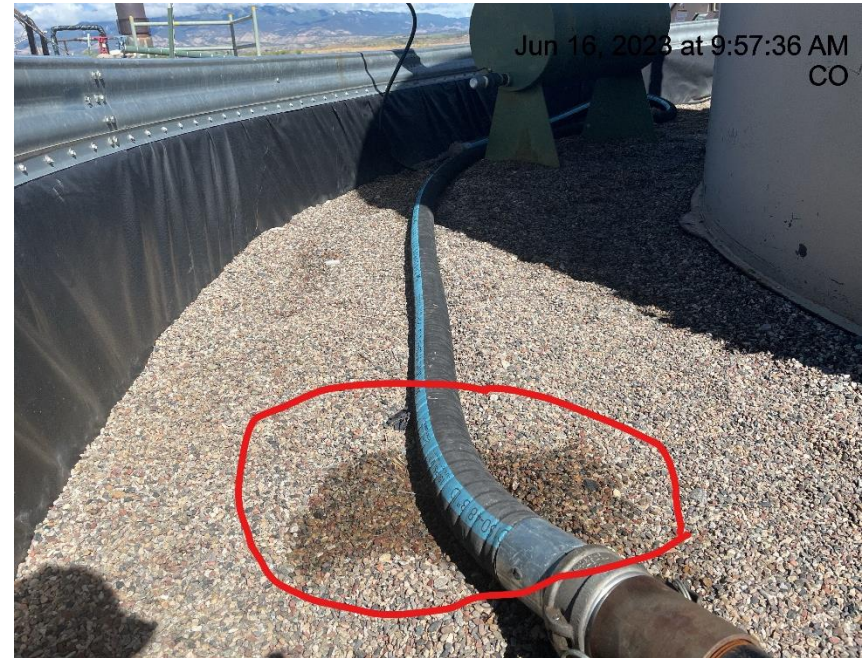
Photo # 745 Stained gravel in secondary containment
