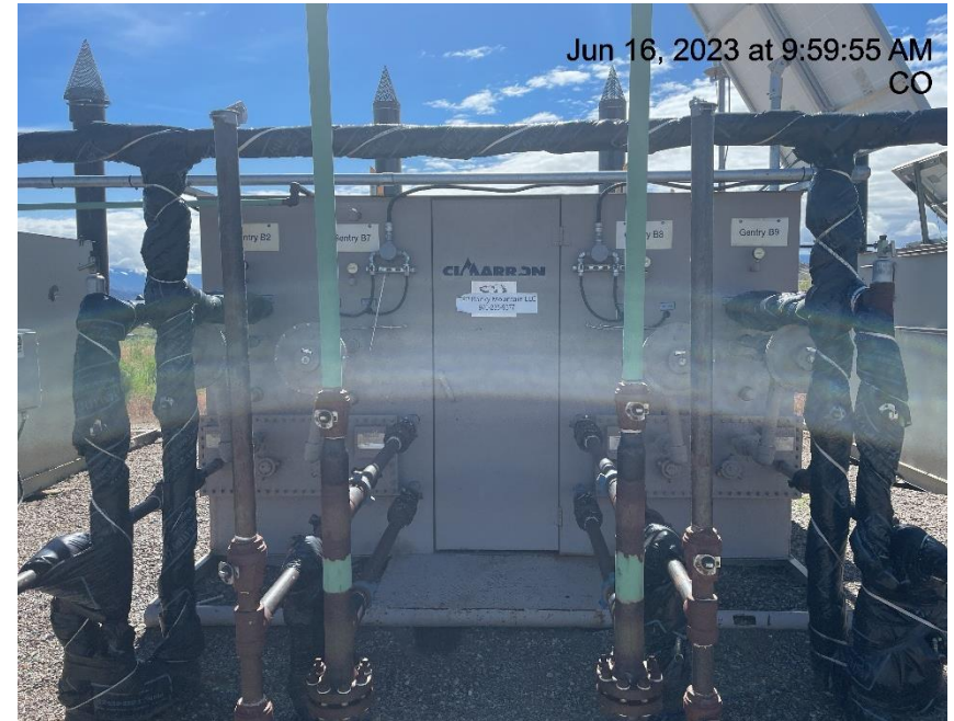
Photo # 751 Meter calibration info not conspicuously posted
