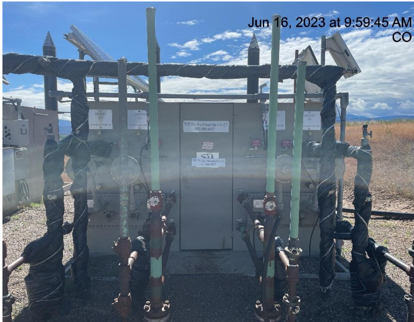
Photo # 750 Meter calibration info not conspicuously posted
