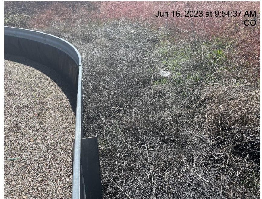
Photo # 741 Debris around secondary containment
