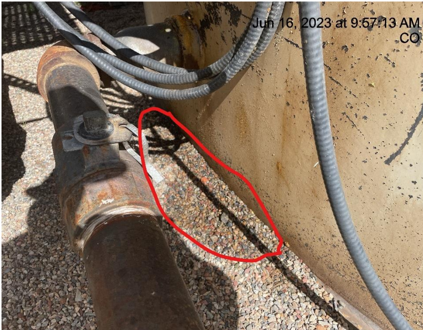
Photo # 744 Stained gravel in secondary containment
