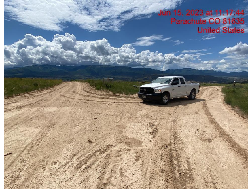
Insufficient Vehicle Tracking BMPs at Location Entrance/Exit – Photo #04550
