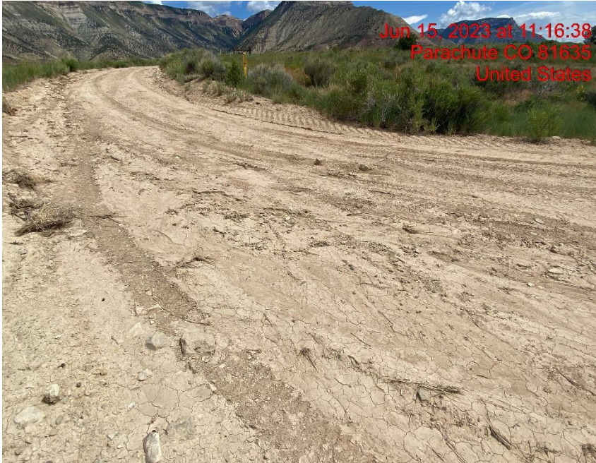
Access Road Lacks Stabilization – Photo #04549
