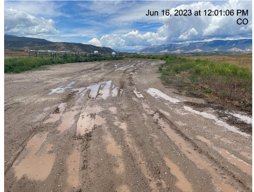
Photo # 959 Lack of stabilization/compaction
