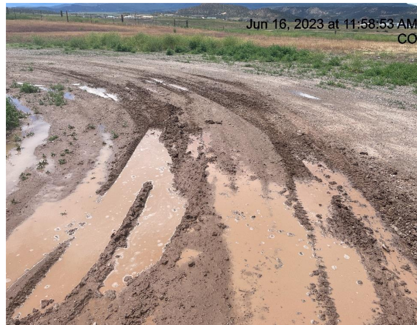
Photo # 950 Lack of stabilization/compaction
