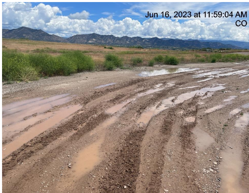
Photo # 951 Lack of stabilization/compaction
