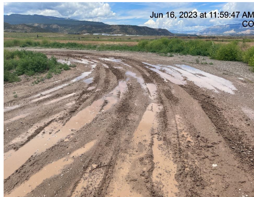
Photo # 953 Lack of stabilization/compaction
