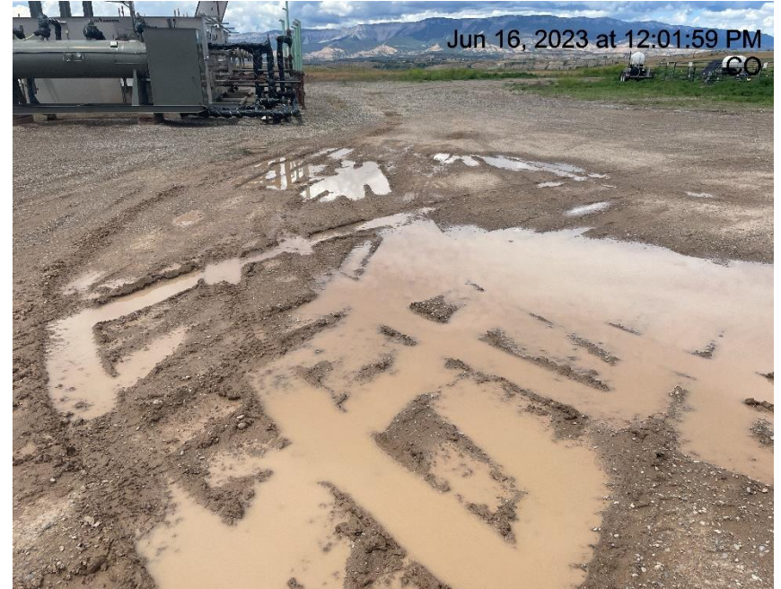
Photo # 962 Lack of stabilization/compaction
