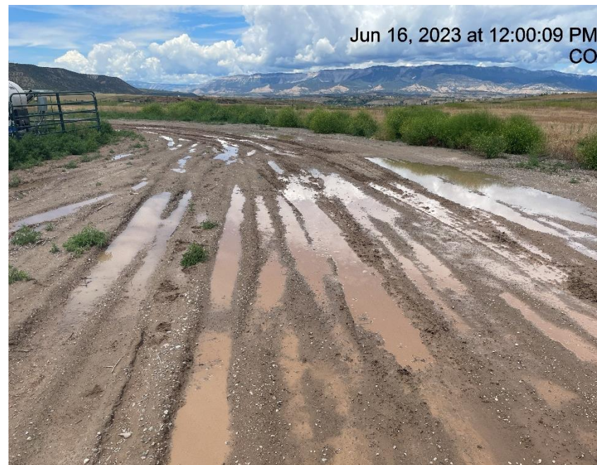
Photo # 955 Lack of stabilization/compaction
