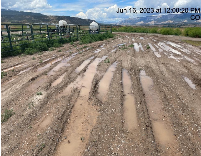
Photo # 956 Lack of stabilization/compaction
