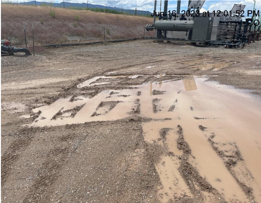
Photo # 961 Lack of stabilization/compaction
