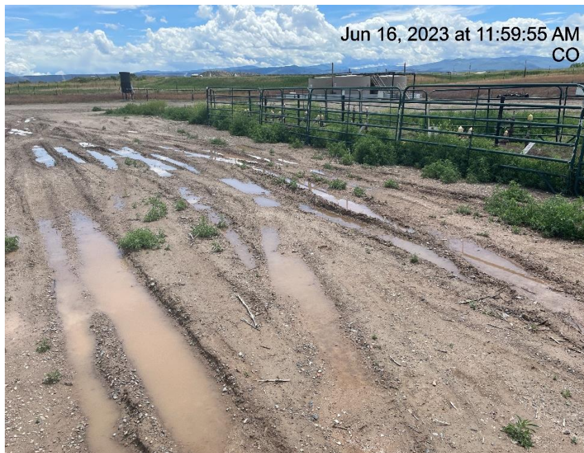
Photo # 954 Lack of stabilization/compaction
