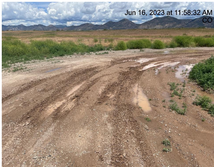
Photo # 949 Lack of stabilization/compaction
