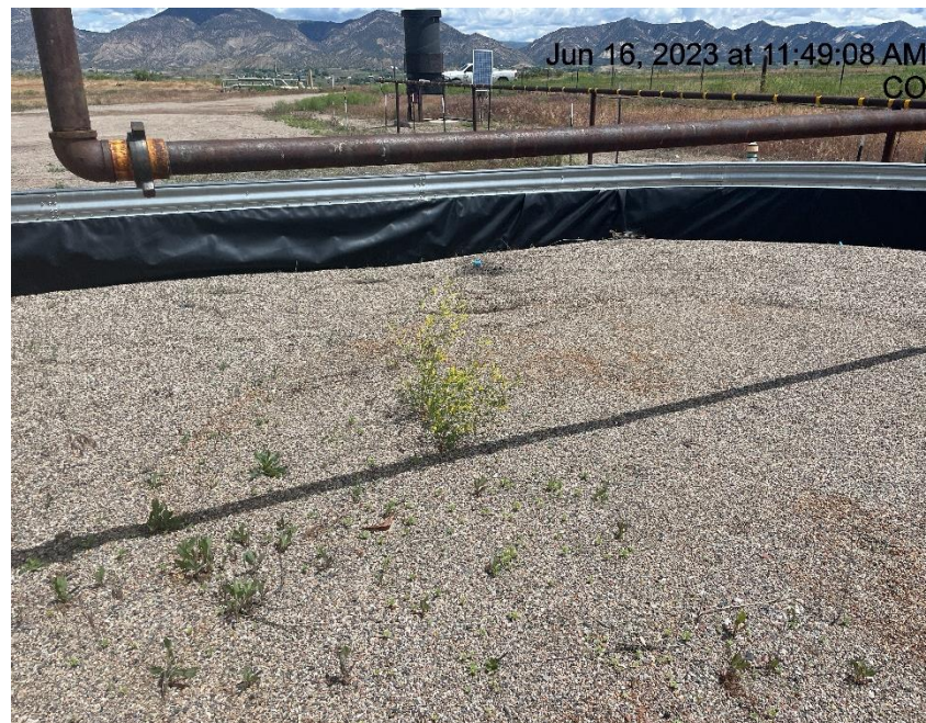
Photo # 927 Weeds/undesirable plant species in secondary containment
