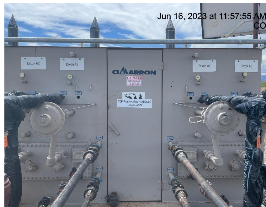
Photo # 948 Meter calibration info not conspicuously posted
