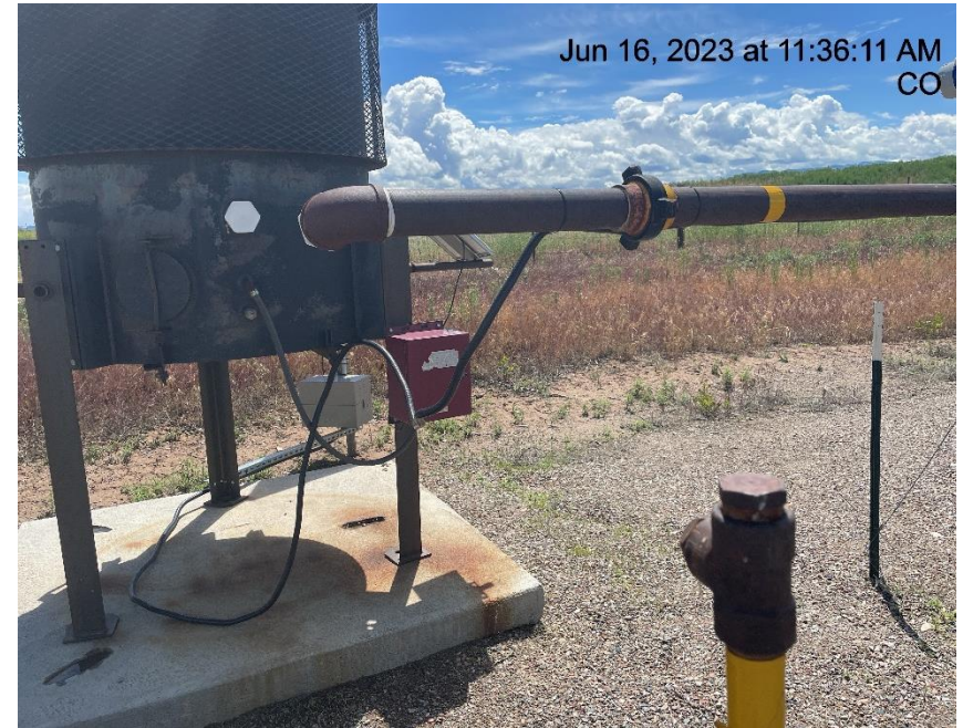
Photo # 921 Unused equipment - ECD is disconnected
