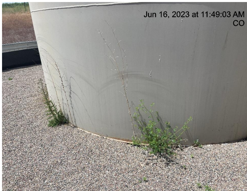
Photo # 926 Weeds/undesirable plant species in secondary containment
