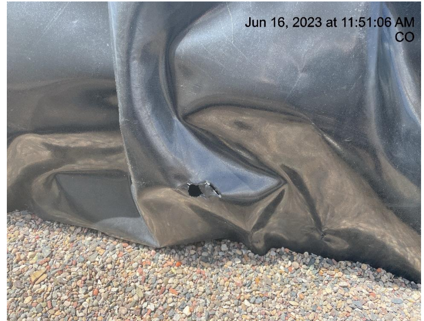
Photo # 935 Hole in liner/liner needs maintenance
