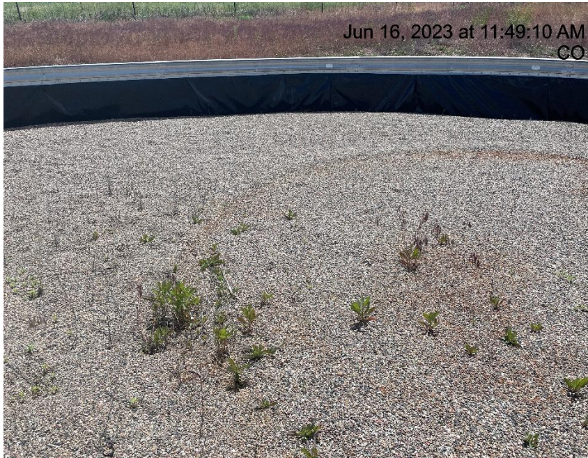
Photo # 928 Weeds/undesirable plant species in secondary containment
