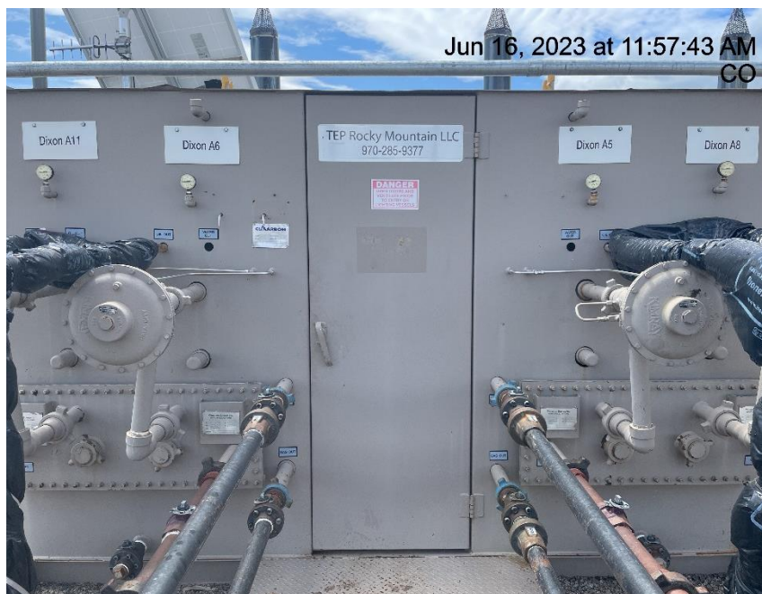
Photo # 947 Meter calibration info not conspicuously posted
