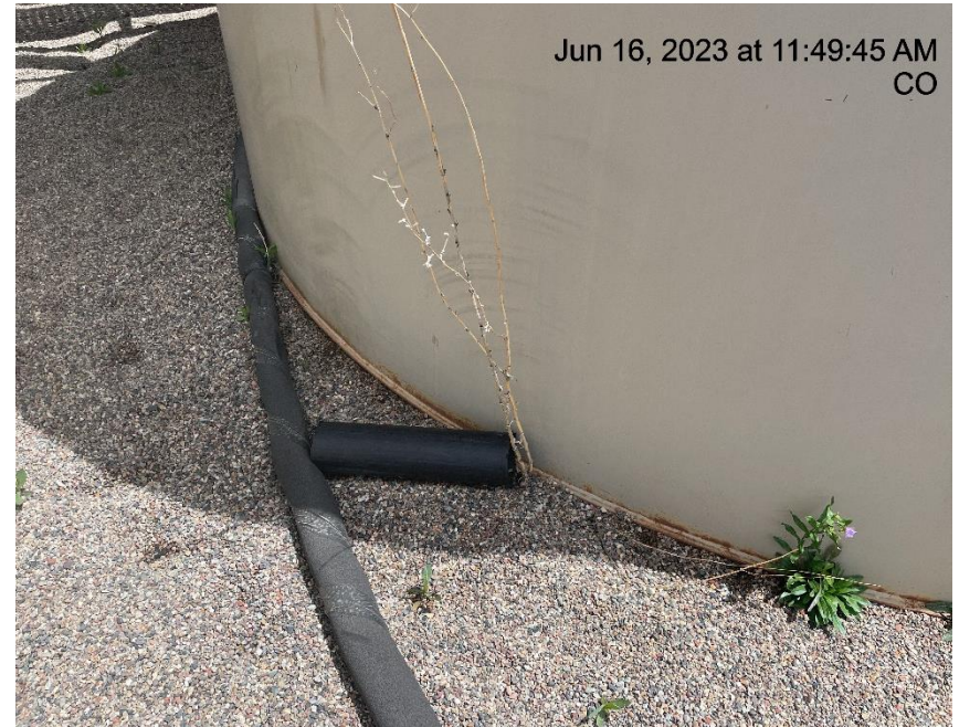
Photo # 929 Weeds/undesirable plant species in secondary containment
