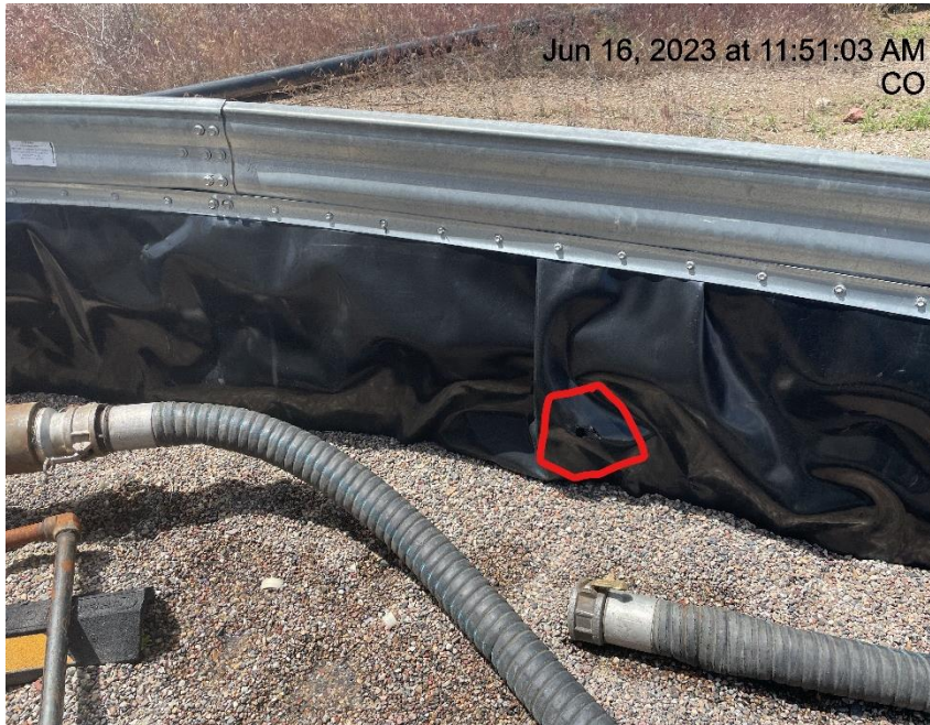
Photo # 934 Hole in liner/liner needs maintenance
