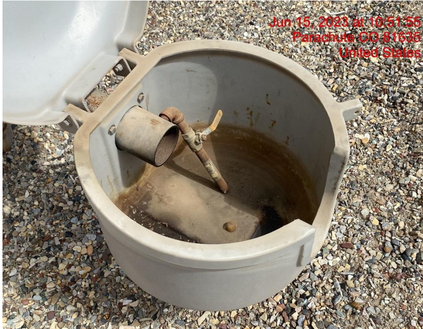
Open-Ended Line on Condensate Tank – Photo #04512
