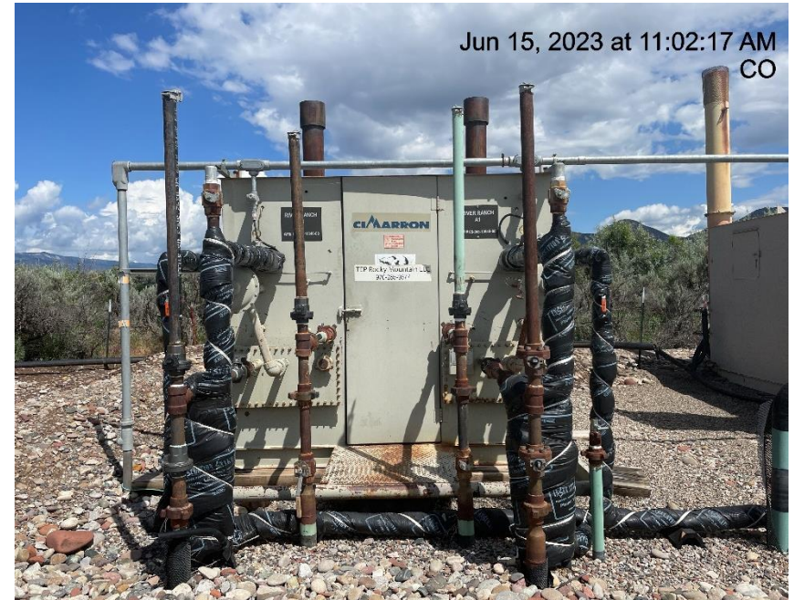
Photo # 616 Meter calibration info not conspicuously posted
