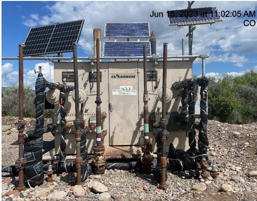
Photo # 615 Meter calibration info not conspicuously posted
