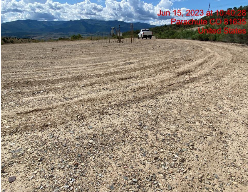
Location Lacks Stabilization – Photo #04497
