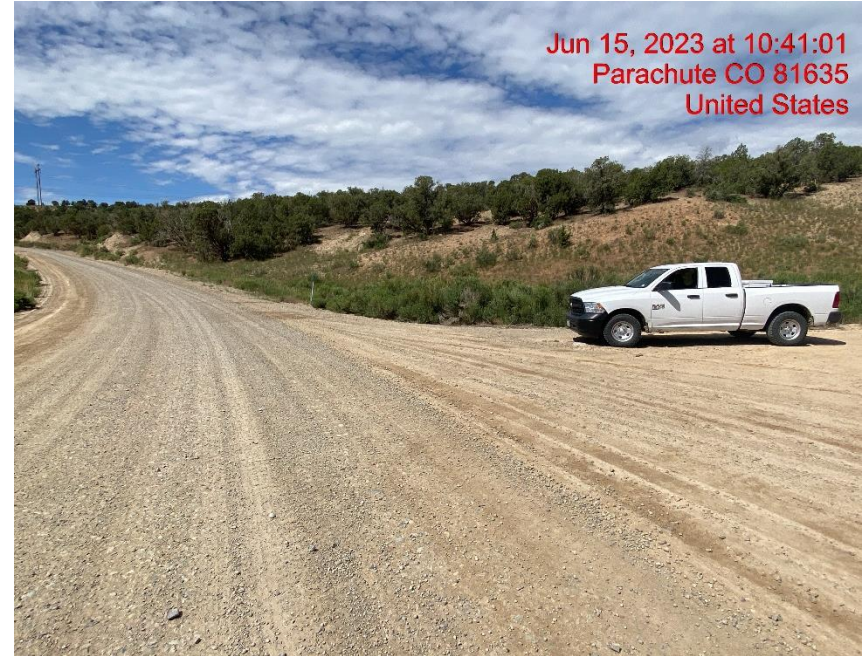
Insufficient Vehicle Tracking BMPs at Location Entrance/Exit – Photo #04498
