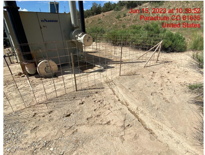
Rill Erosion Transporting Sediment onto Location – Photo #04491
