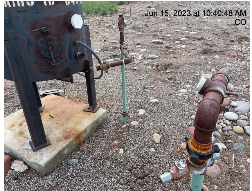
Photo # 595 Unused equipment - ECD is disconnected
