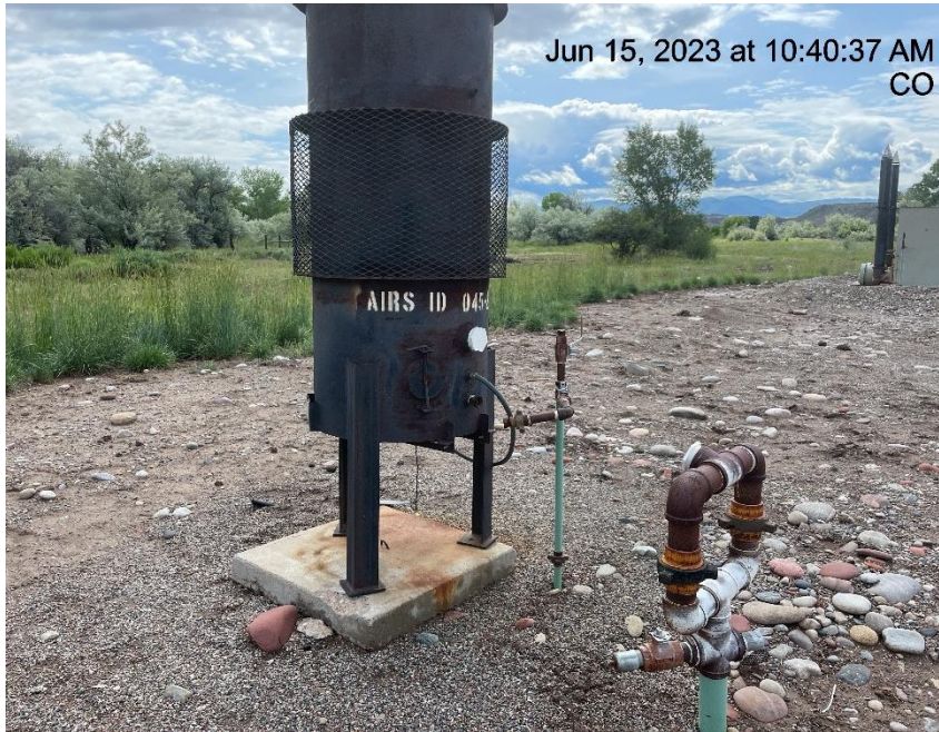
Photo # 594 Unused equipment - ECD is disconnected
