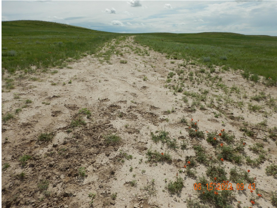
Photo 1. Photo taken from the western access road, facing East. Photo illustrates the access road has partial establishment of desirable vegetation but there is evidence of erosion.
