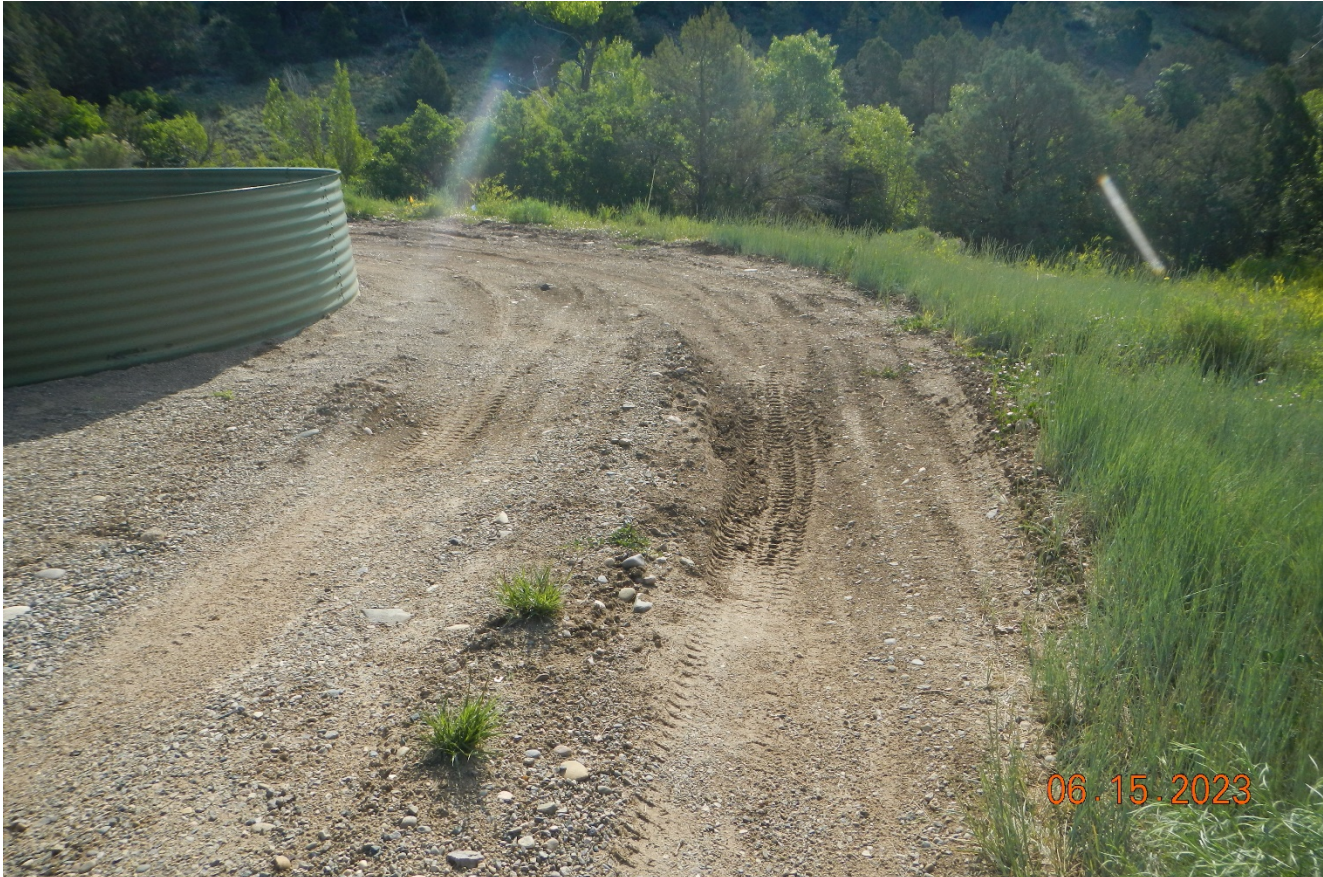
Photo 7. There is vehicle ruts where stormwater accumulates which need to be repaired.
