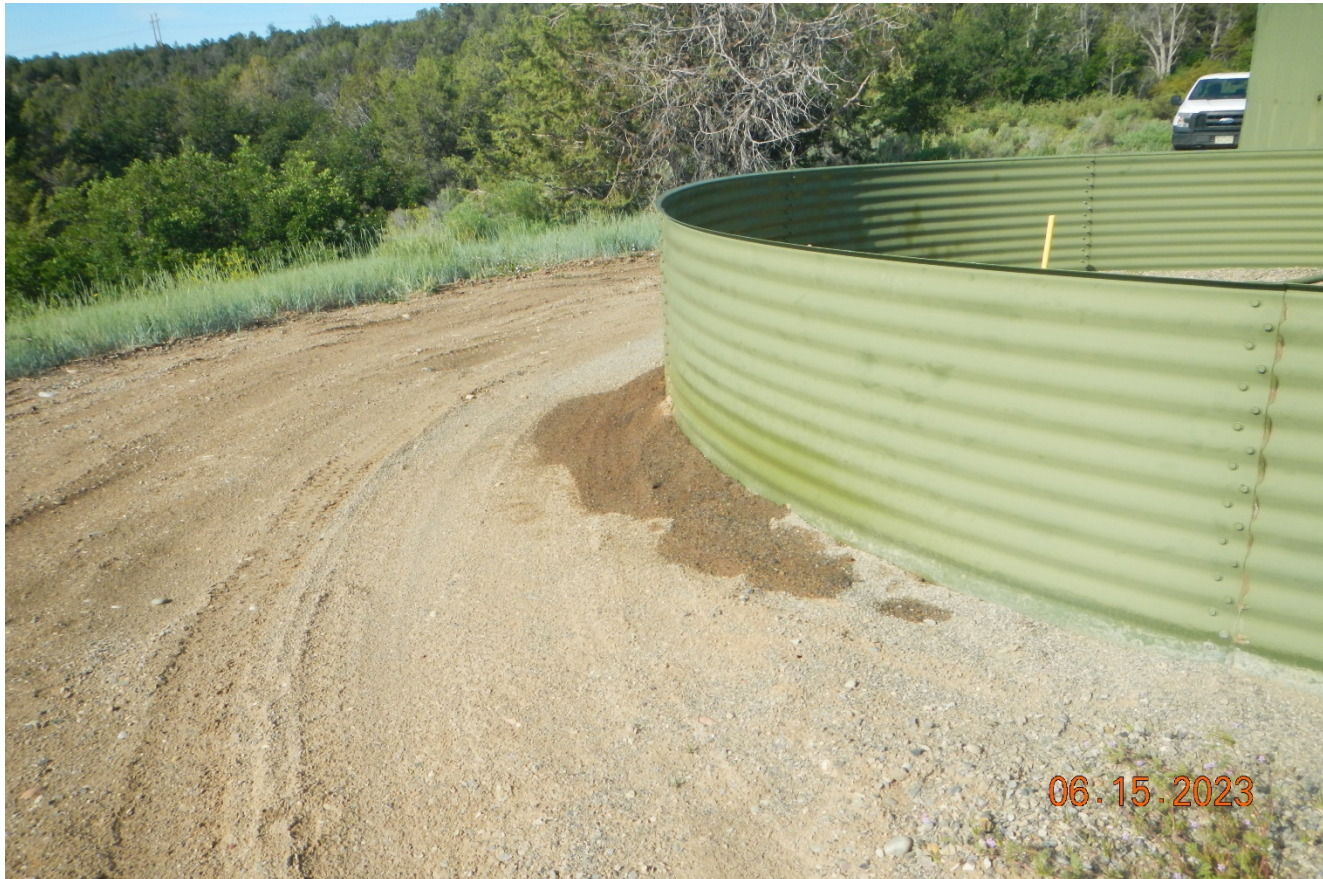
Photo 5. There is oil stained soils outside of containment at the buried tank.
