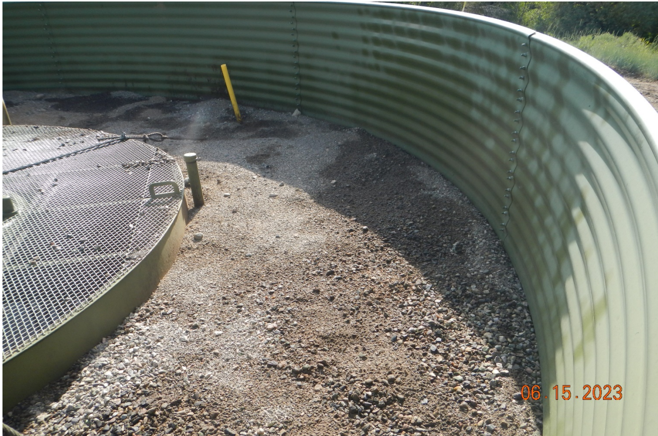
Photo 6. There are stain soils inside containment that need to be cleaned up.
