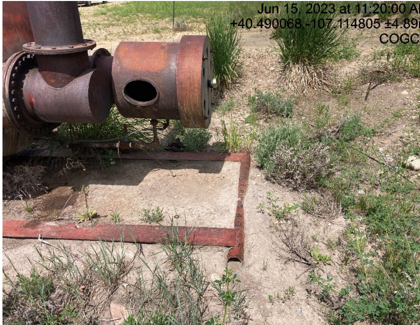
Weeds around production equipment and open hole for wildlife to enter.
