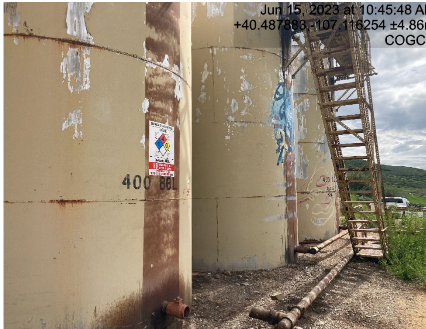
Open load line, debris and tanks lacking signage
