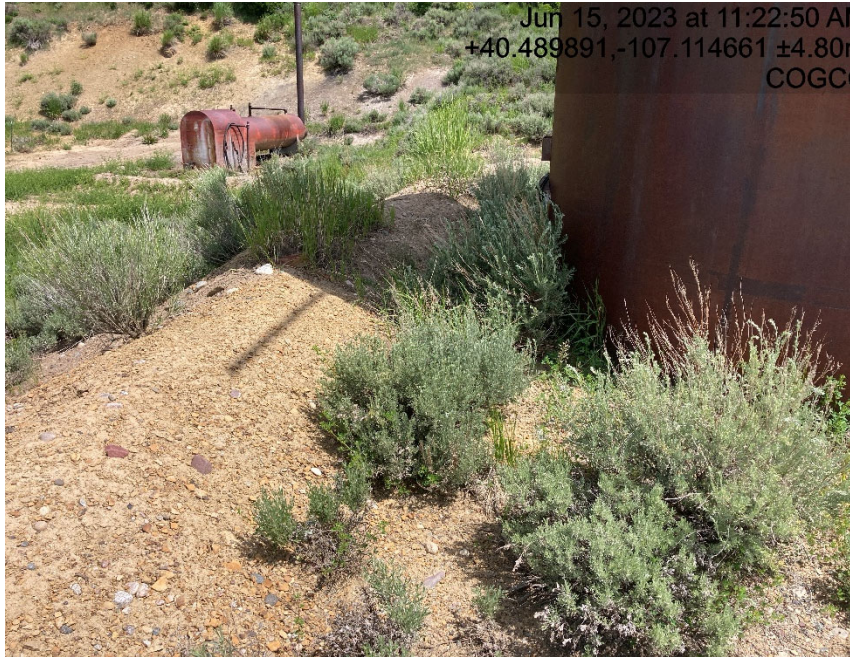
Weeds around equipment and in secondary containment
