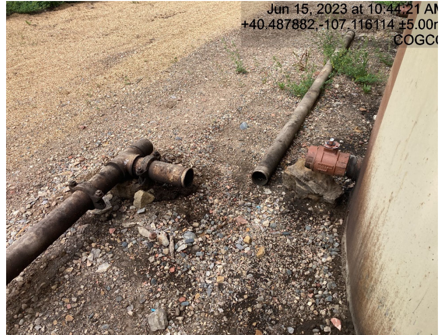
Debris and open load line
