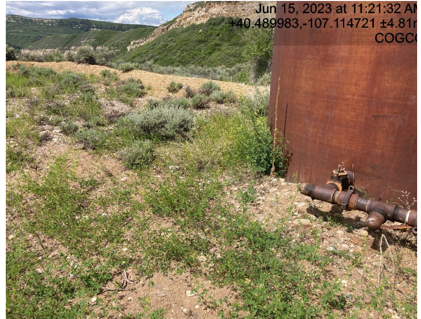
Weeds around equipment and in secondary containment
