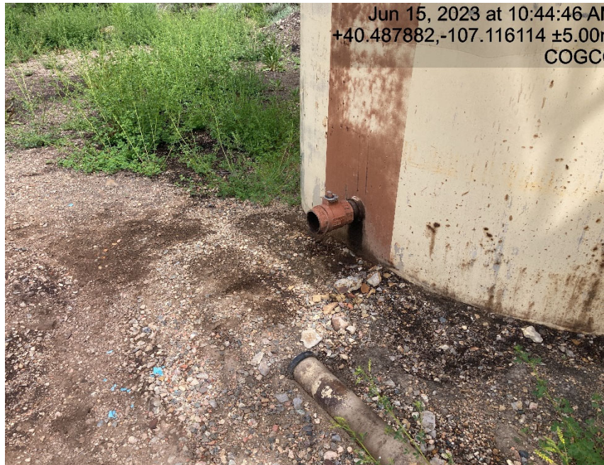
Staining, open ended load line on tank and weeds in secondary containment
