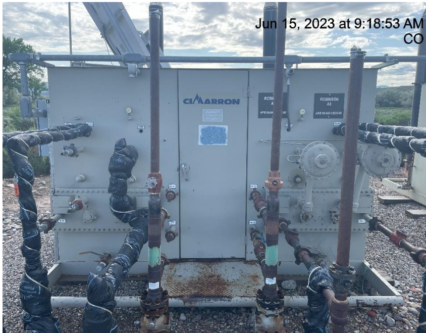
Photo # 494 Meter calibration info not conspicuously posted
