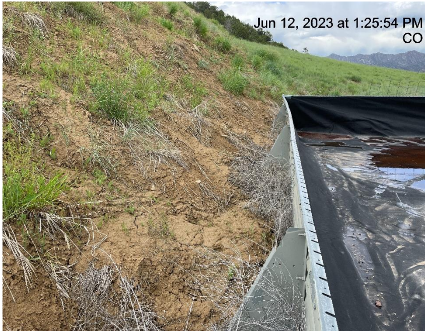
Photo # 230 Erosion/sediment encroaching on equipment
