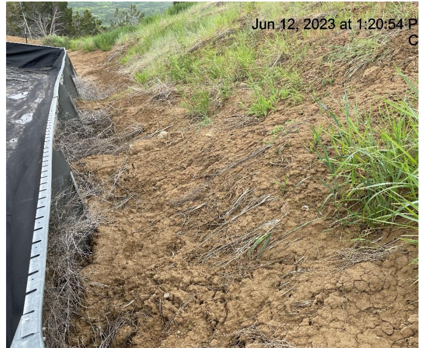
Photo # 217 Erosion/sediment encroaching on equipment
