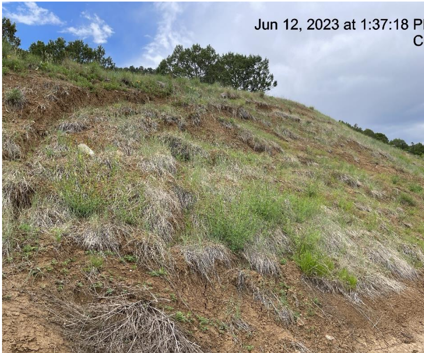
Photo # 259 Lack of stabilization on cut slope
