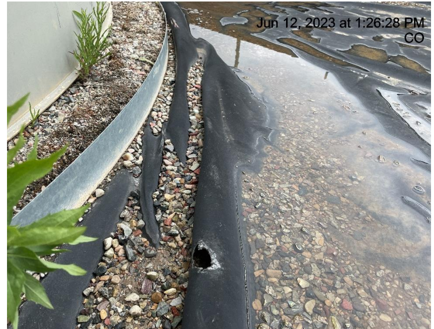
Photo # 232 Hole in base of liner/containment needs maintenance
