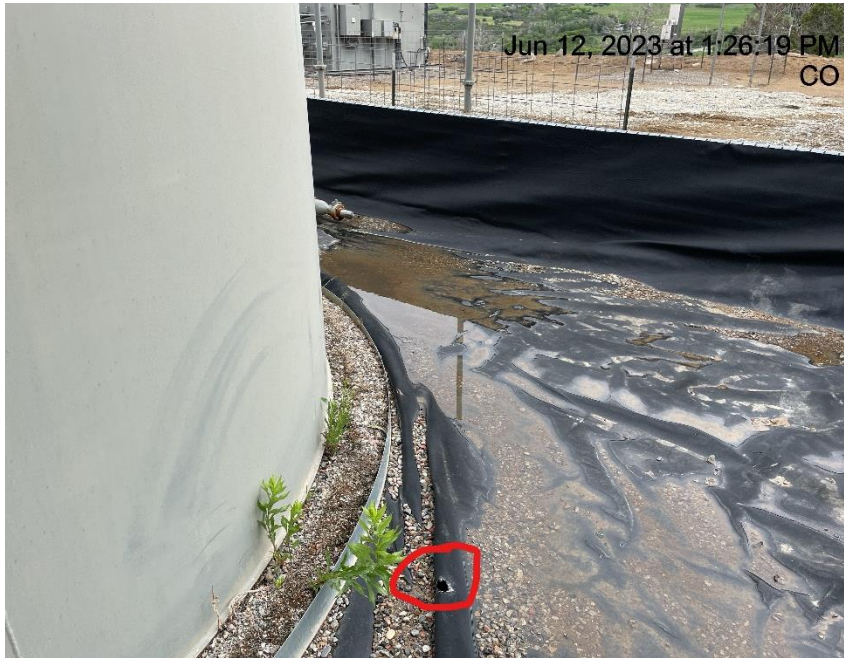
Photo # 231 Hole in base of liner/containment needs maintenance
