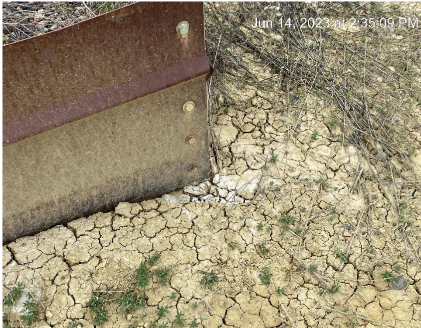
Leaking containment
