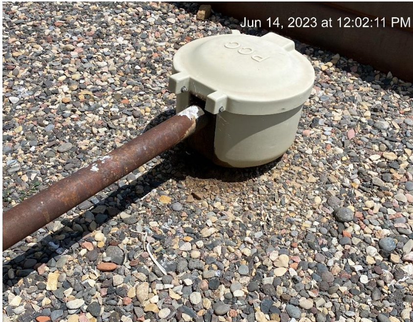
Loadline pot staining and stained soil
