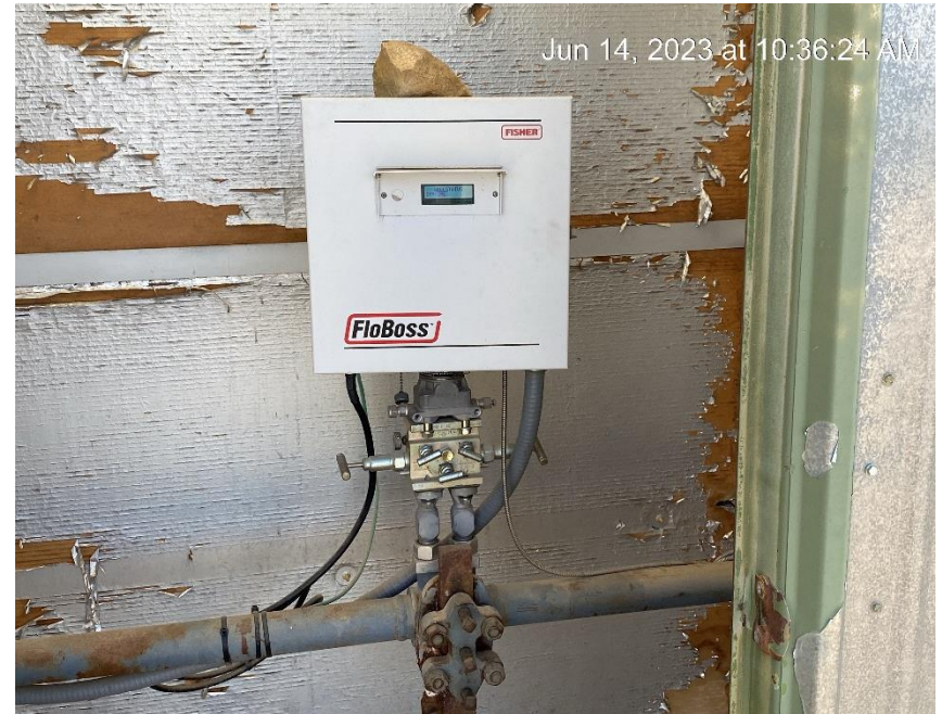
No visible display of gas meter calibration
