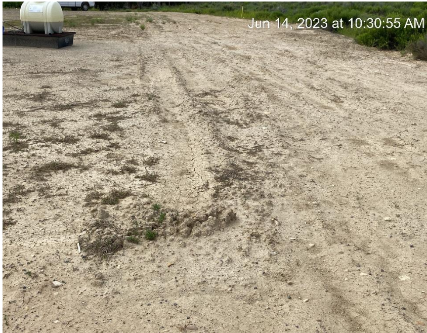
Lack of stabilization. Vehicle tracking.
