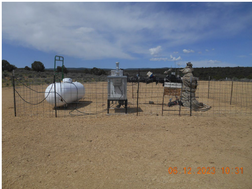
Injection wellhead & line heater
