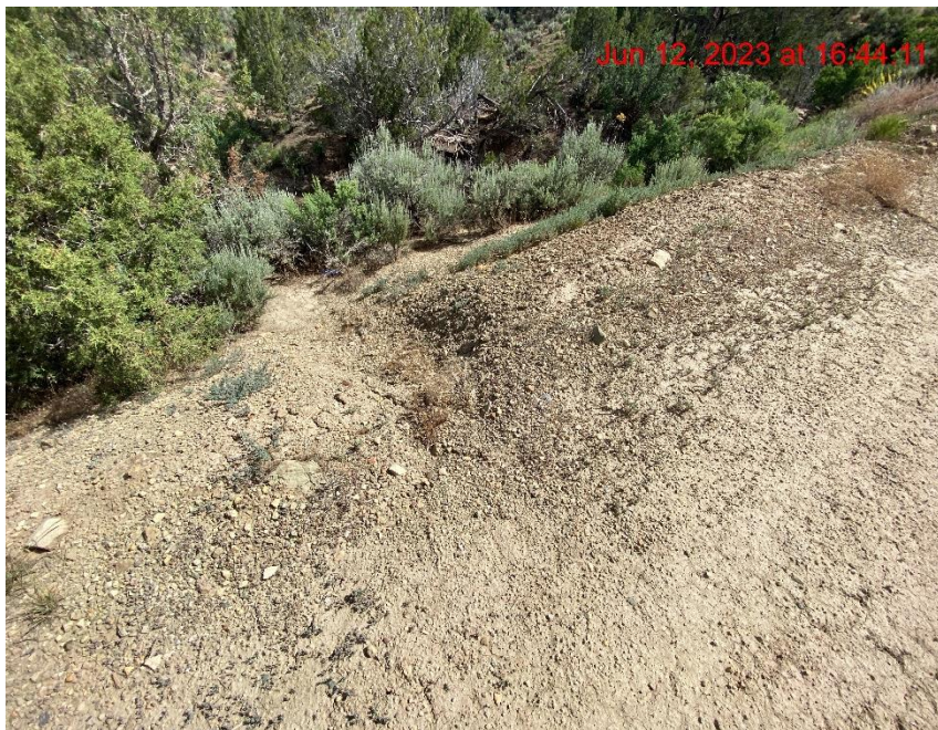
Rill Erosion Transporting Sediment from Access Road to Drainage Ditch – Photo #04399
