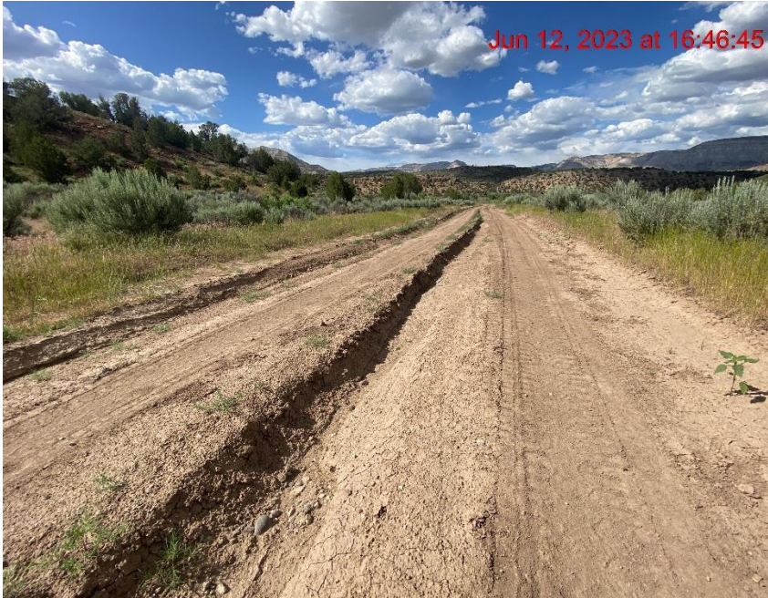
Access Road Lacks Stabilization – Photo #04401
