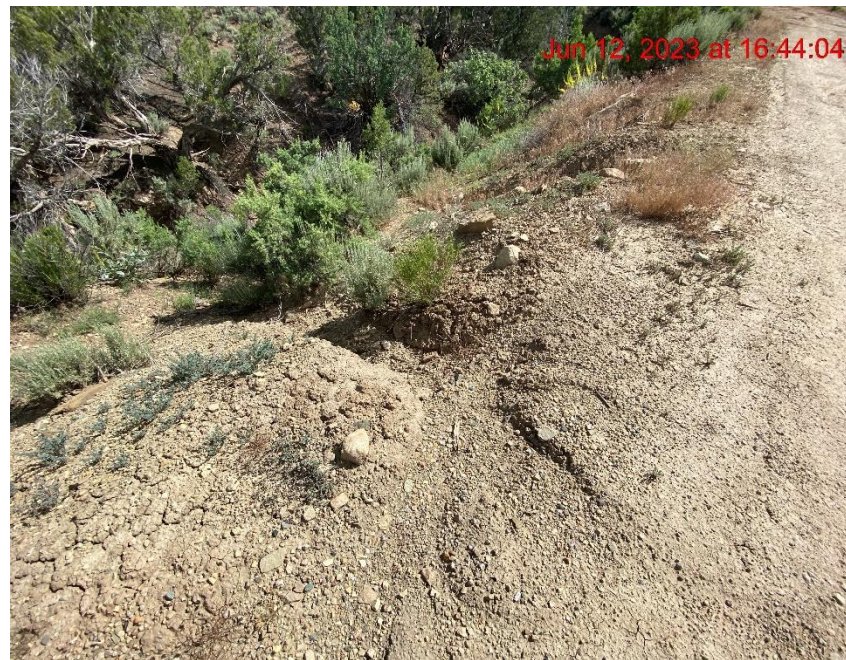
Rill Erosion Transporting Sediment from Access Road to Drainage Ditch – Photo #04398
