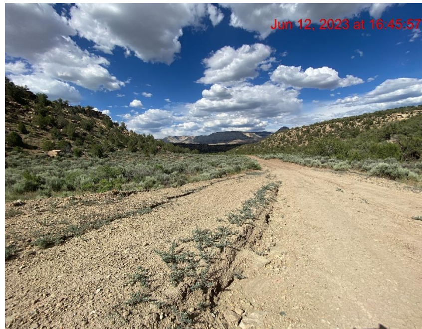
Access Road Lacks Stabilization – Photo #04400
