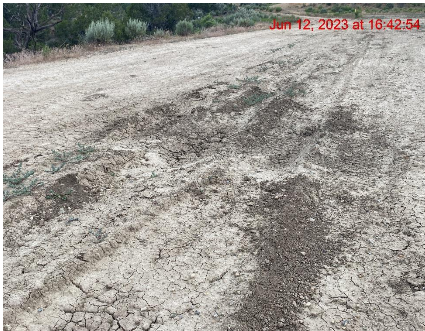
Location Lacks Stabilization – Photo #04393
