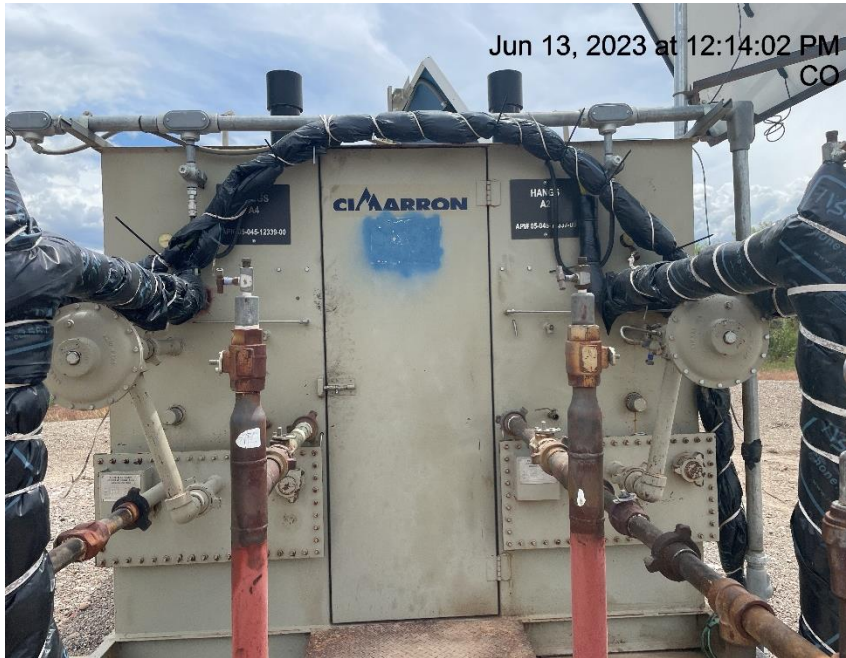
Photo # 347 Meter calibration info not conspicuously posted
