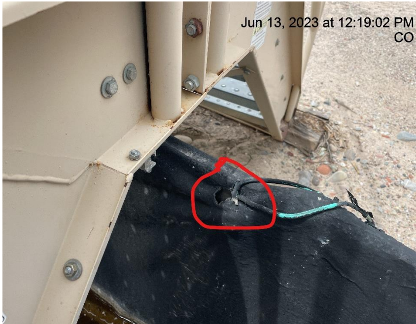
Photo # 355 Containment needs maintenance
