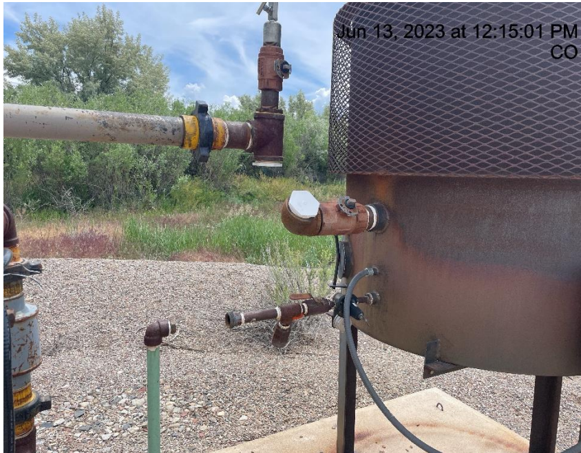
Photo # 349 Unused Equipment – ECD is disconnected & not operational
