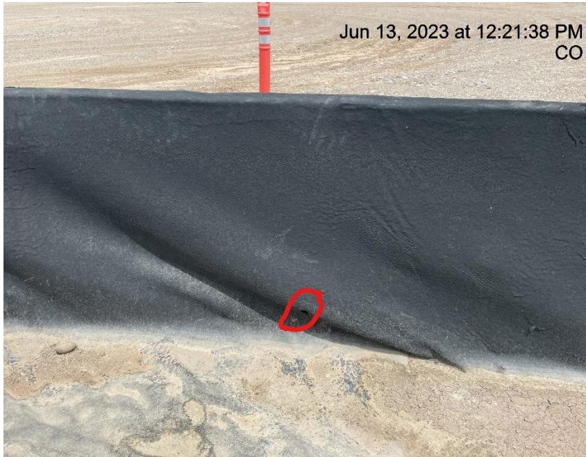
Photo # 358 Containment needs maintenance
