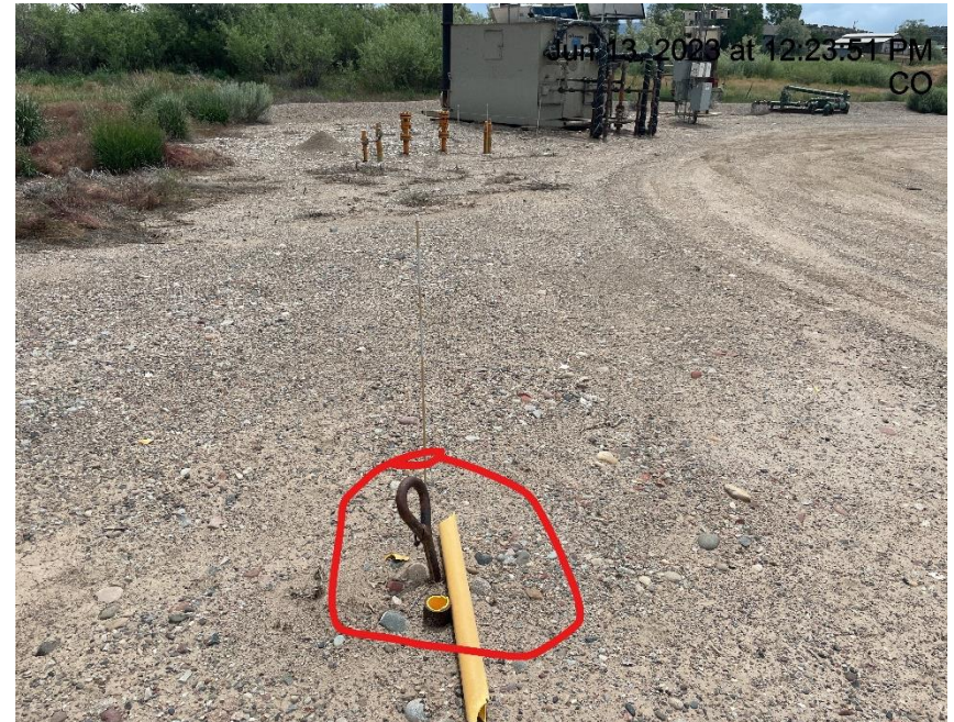
Photo # 362 Improperly marked deadman
