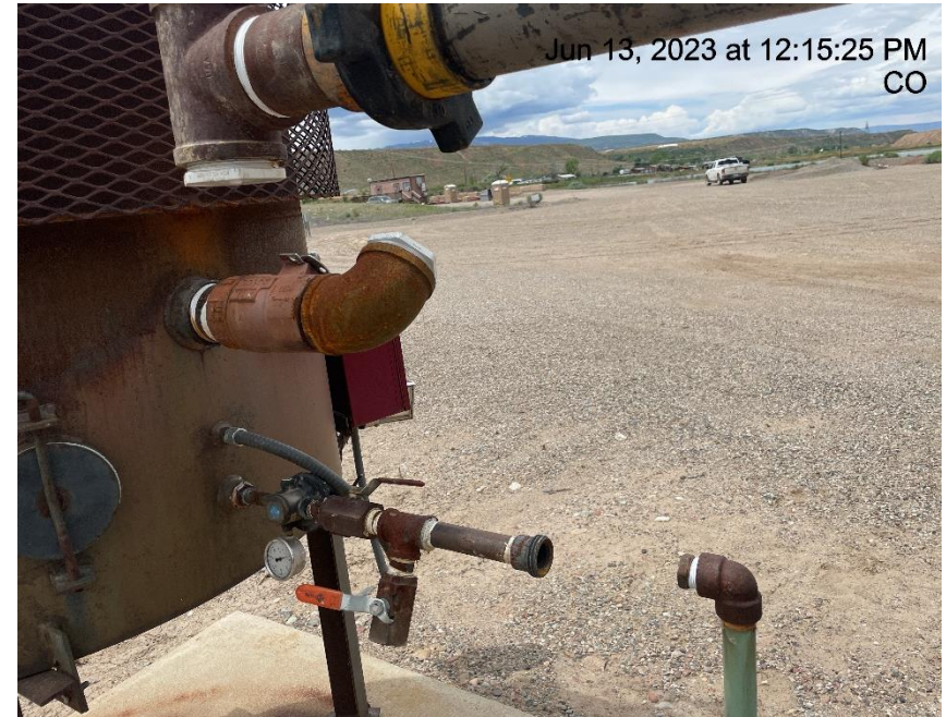
Photo # 350 Unused Equipment – ECD is disconnected & not operational
