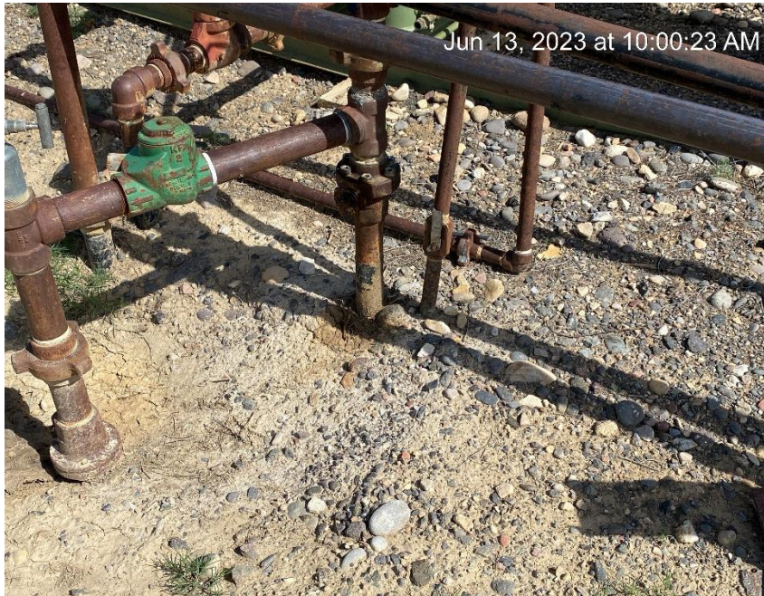
Leaking line and stained soil
