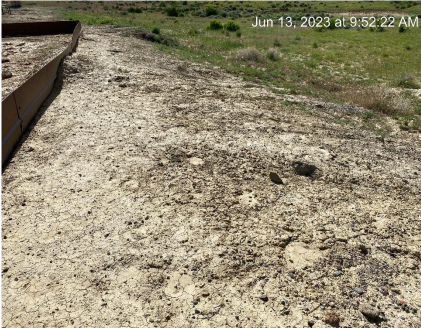
Erosion and sediment migration from location
