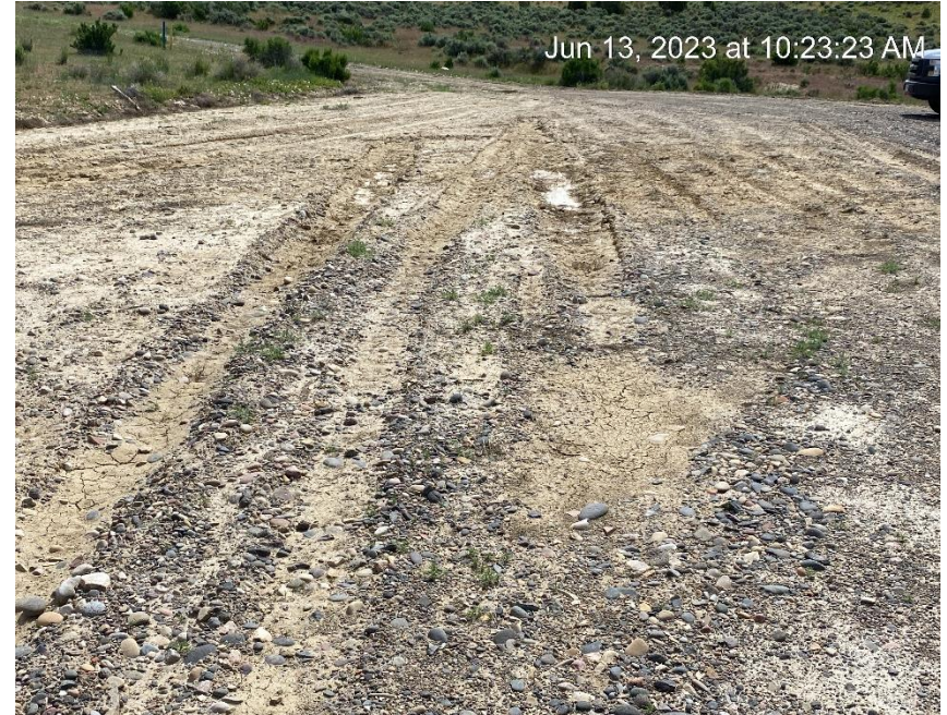
Lack of stabilization and vehicle tracking
