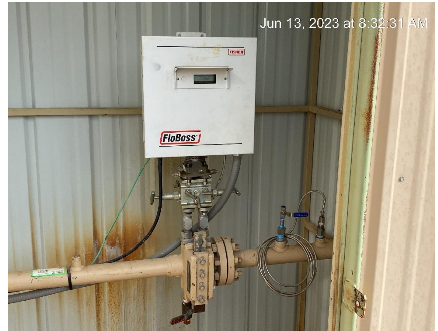
19-22D gas meter calibration not visibly displayed
