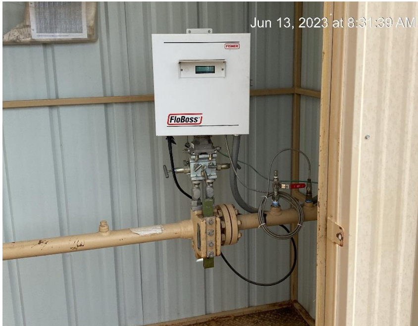
19-21 gas meter calibration not visibly displayed
