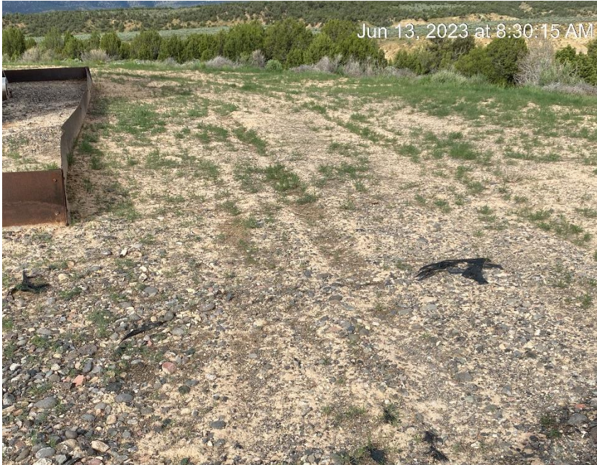
Lack of stabilization. Vehicle tracking
