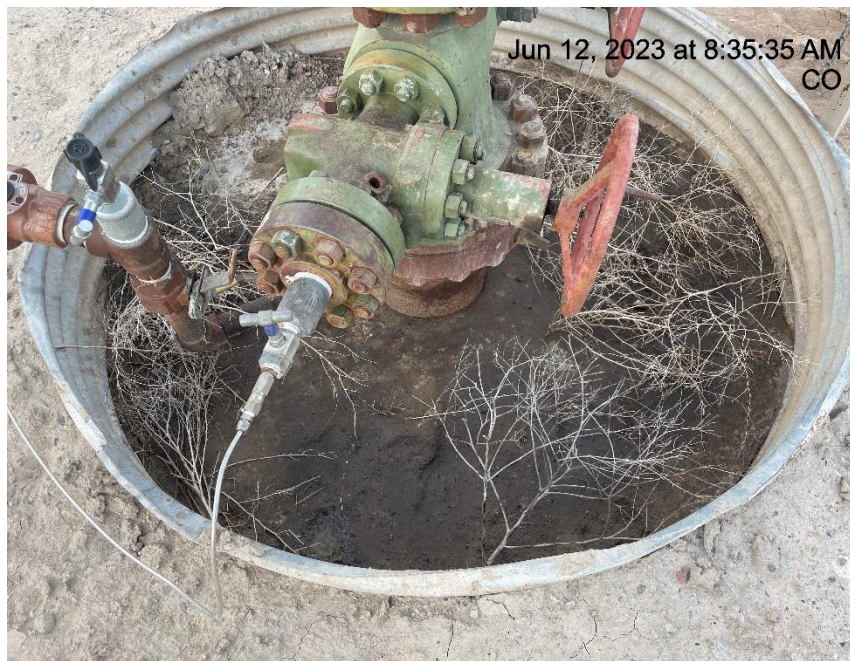
Photo # 72 Stained soils & gravel inside GUCCINI 41C wellhead cellar
