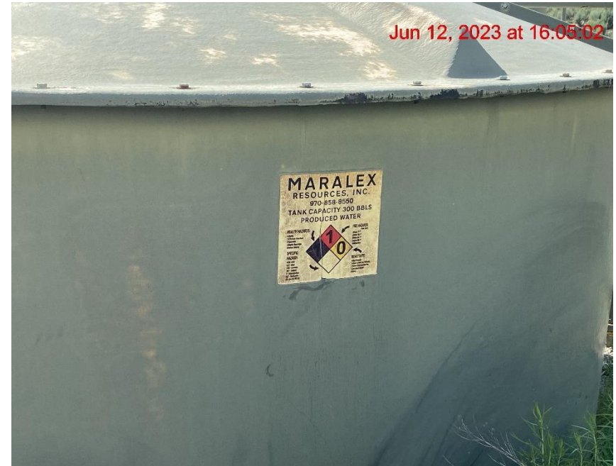
Inaccurate Information on Tank Label – Photo #04341
