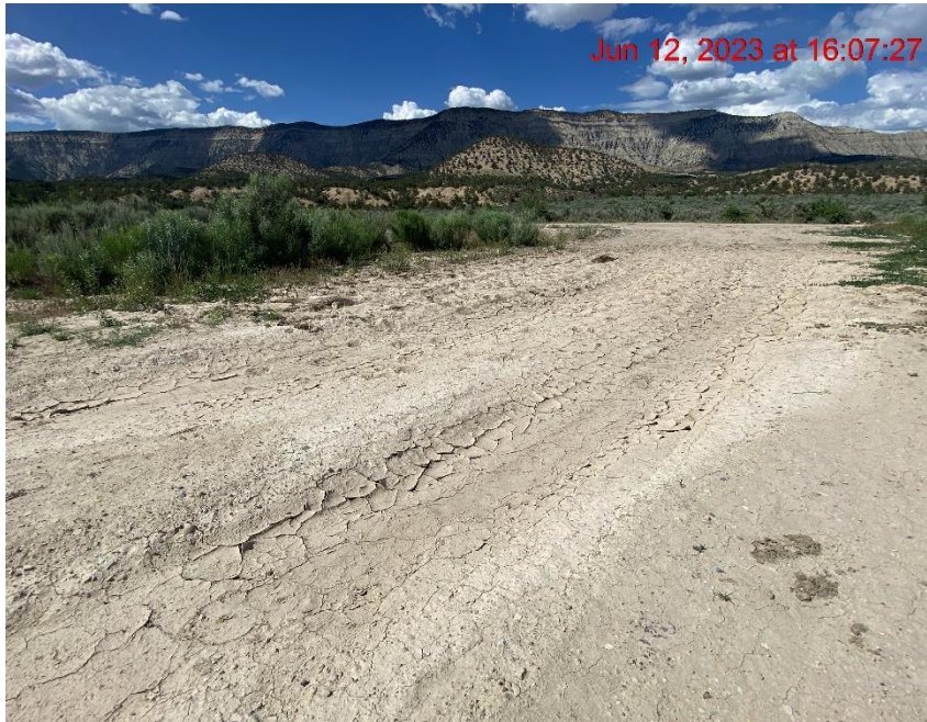
Lack of Stabilization on Access Road – Photo #04346
