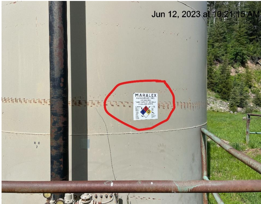
Photo # 130 Tank label has incorrect information
