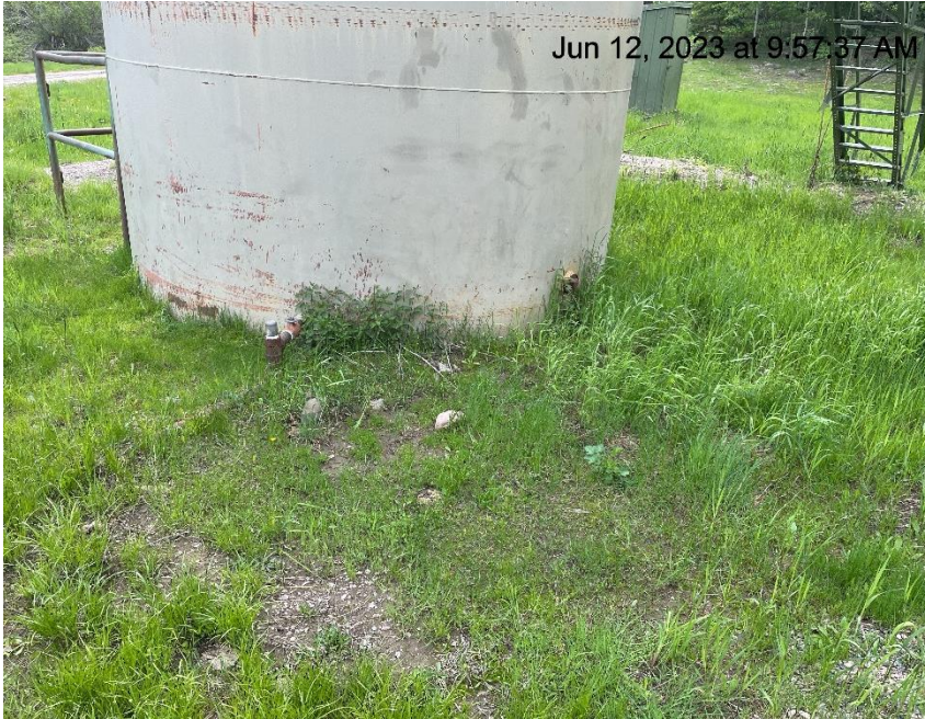
Photo # 98 Weeds/undesirable plant species encroaching on equipment
