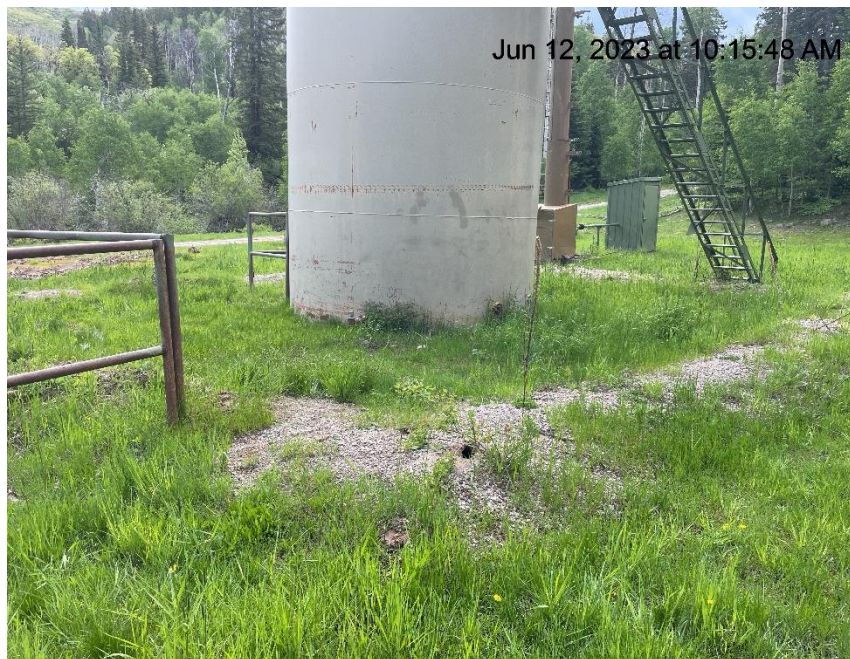
Photo # 126 Secondary containment not sufficient to contain 110% of tank capacity spilled or released materials/containment needs maintenance.
