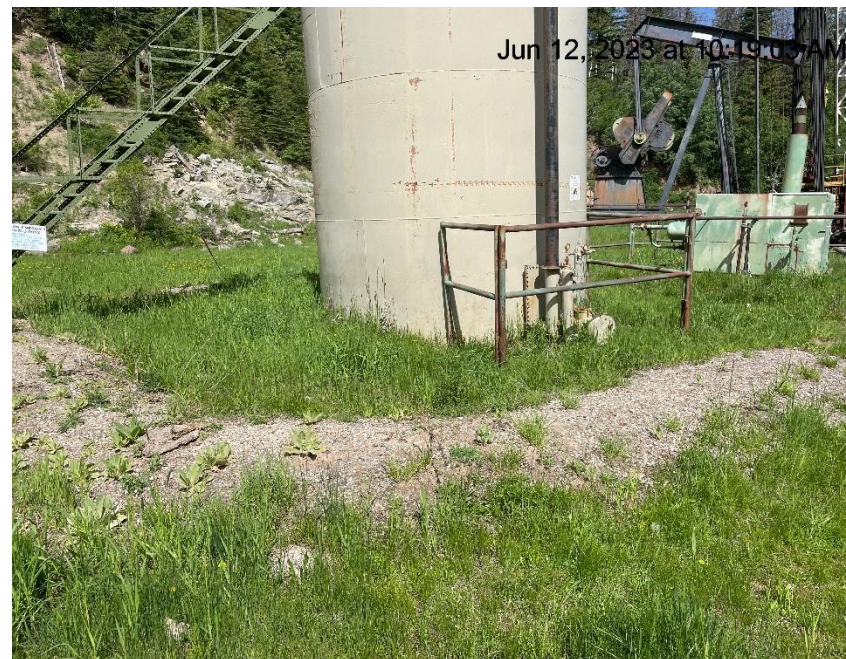
Photo # 128 Secondary containment not sufficient to contain 110% of tank capacity spilled or released materials/containment needs maintenance.
