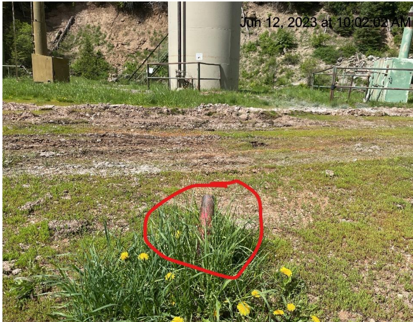
Photo # 109 Improperly marked deadman/anchor
