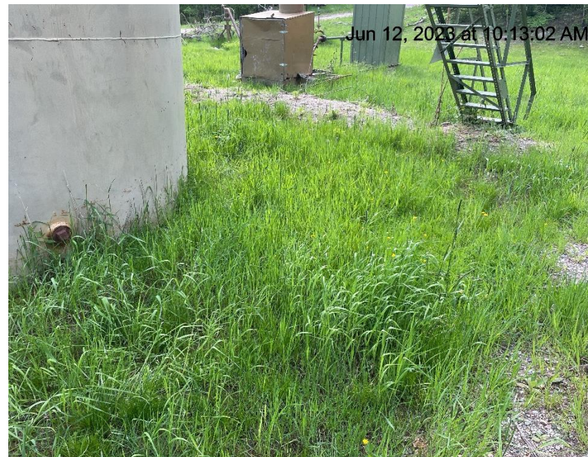
Photo # 123 Secondary containment not sufficient to contain 110% of tank capacity spilled or released materials/containment needs maintenance.
