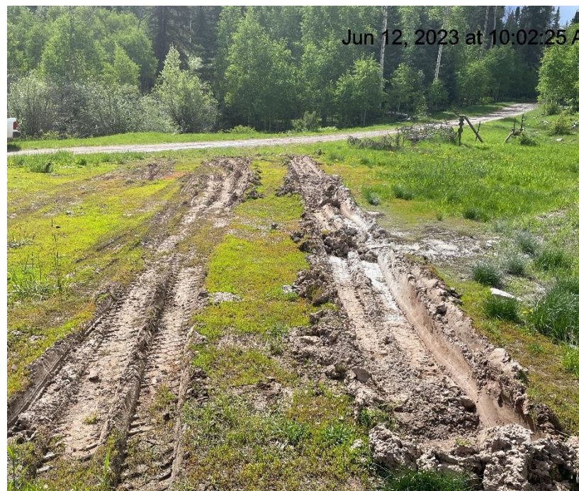
Photo # 110 Lack of stabilization/compaction
