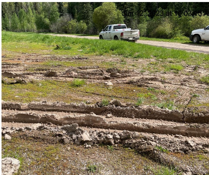
Photo # 114 Lack of stabilization/compaction
