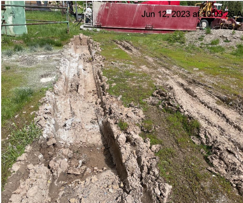
Photo # 116 Lack of stabilization/compaction
