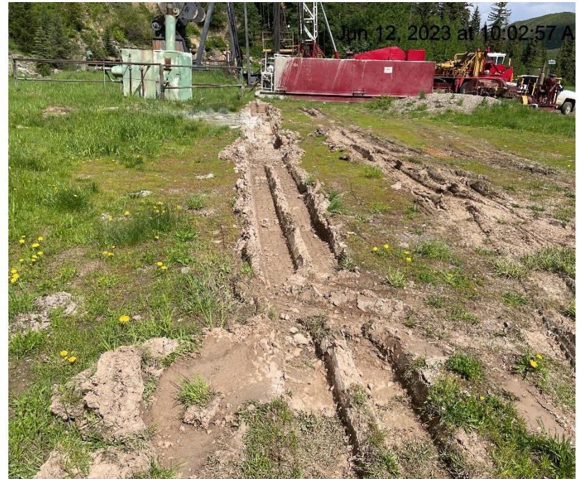
Photo # 112 Lack of stabilization/compaction
