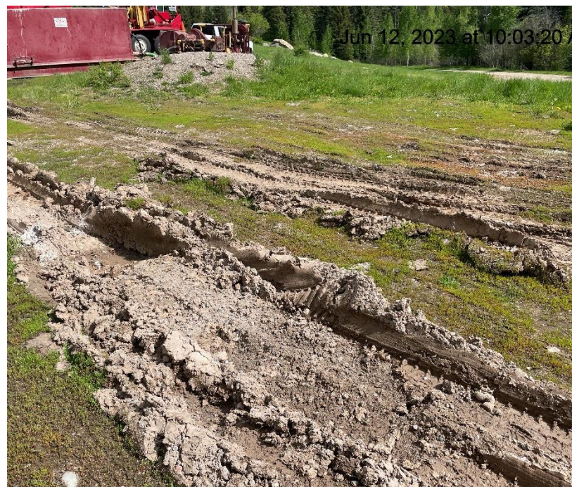
Photo # 115 Lack of stabilization/compaction
