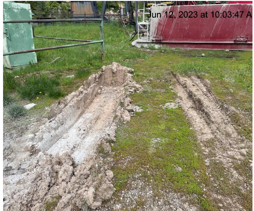
Photo # 118 Lack of stabilization/compaction
