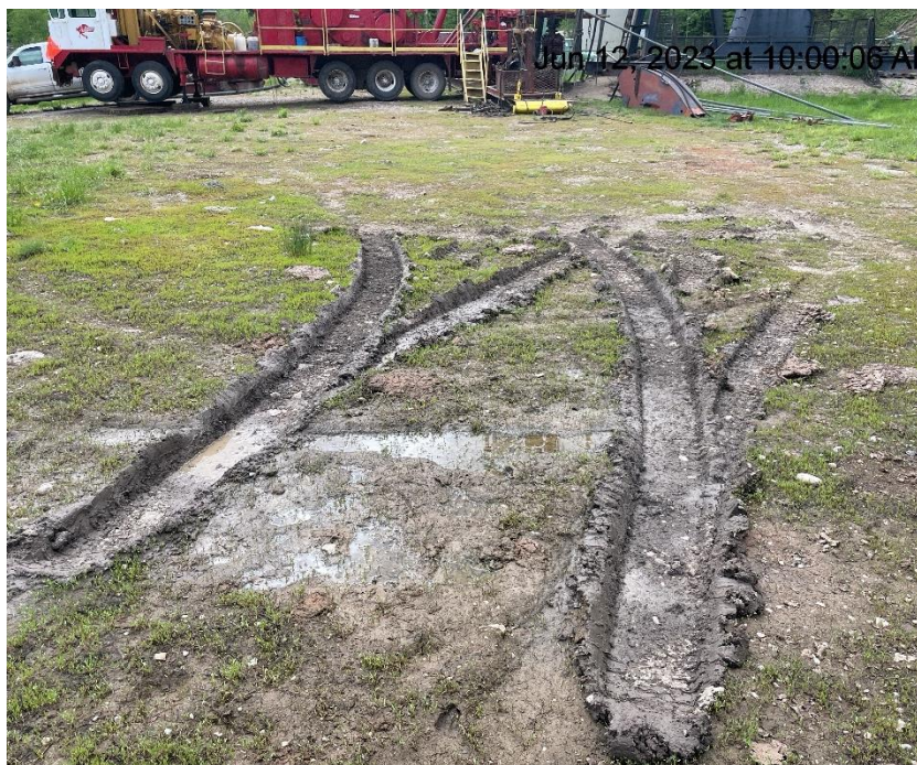
Photo # 102 Lack of stabilization/compaction
