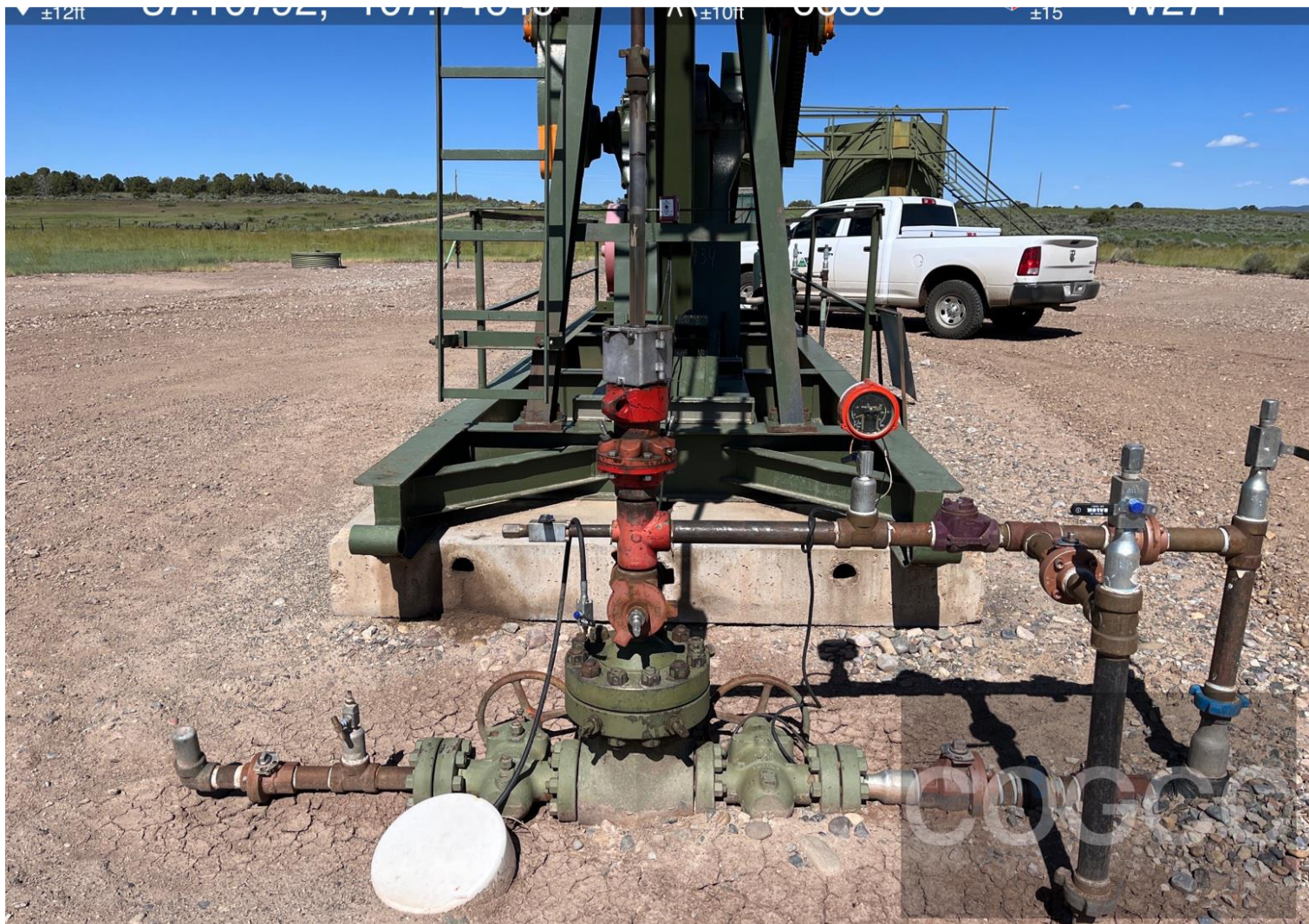
Photo #2 View of the Harmon A2 wellhead assembly.
