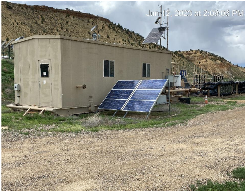
Separator building and flowline manifold
