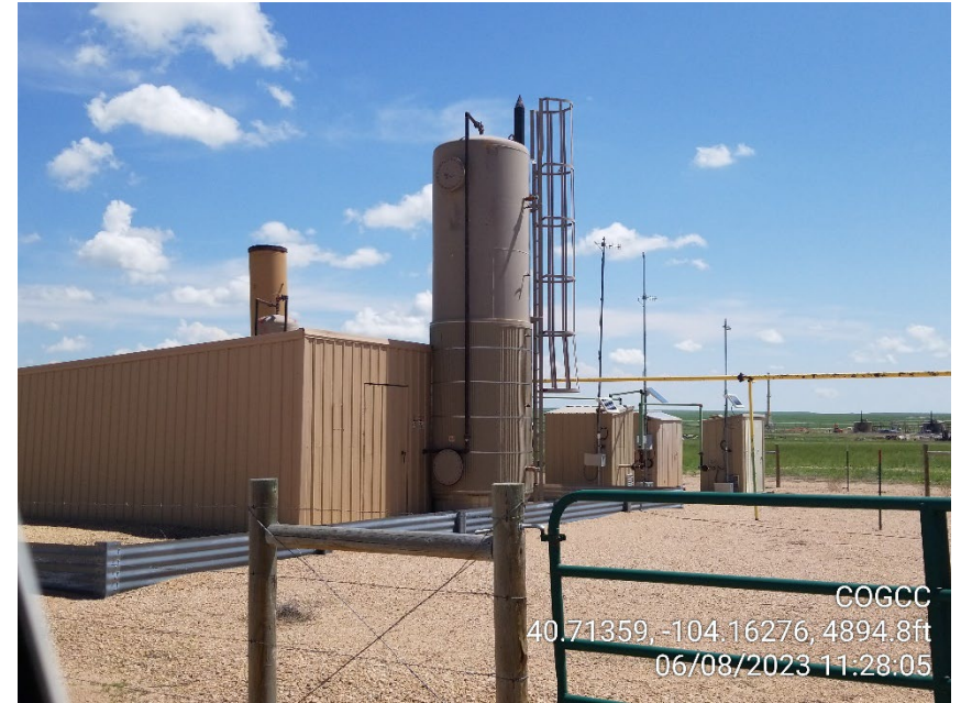
Photo 4 – Heater Treater and Gas Meters
