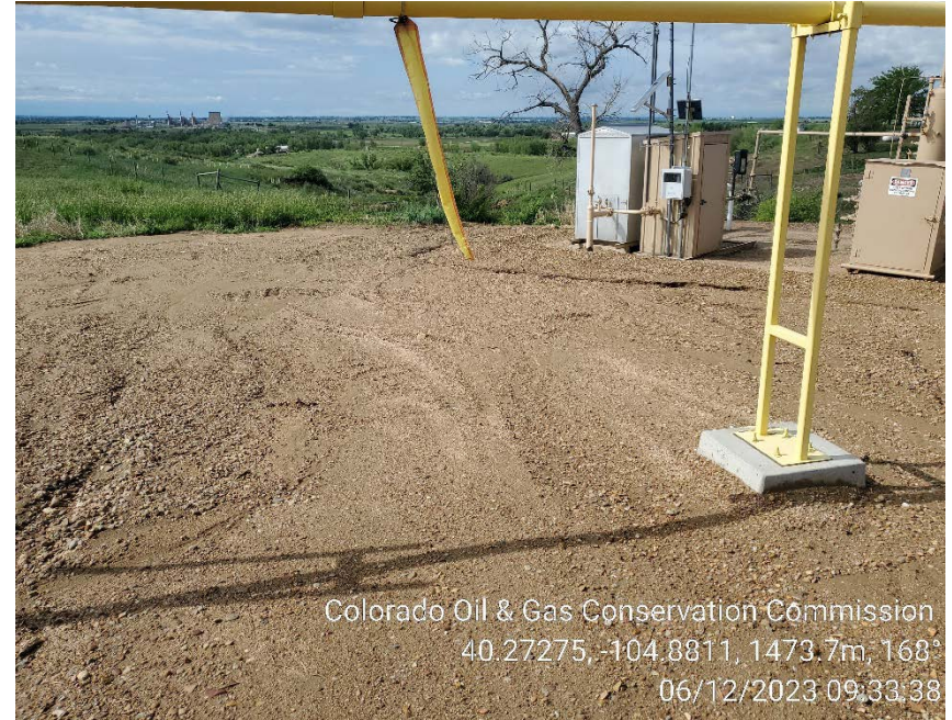
Storm water BMP's on 6/12/2023
