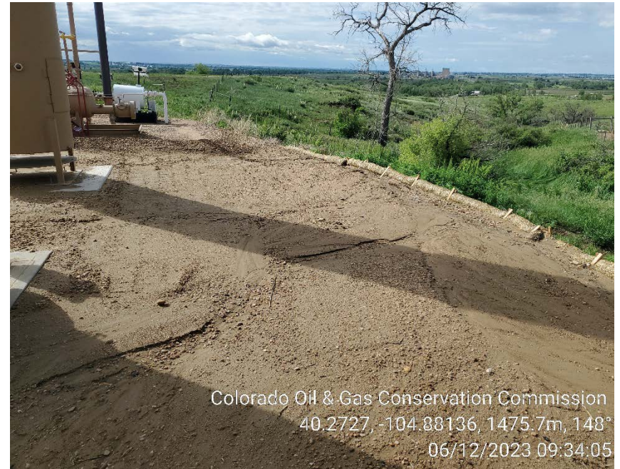
Storm water BMP's on 6/12/2023
