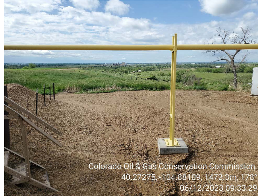
Storm water BMP's on 6/12/2023
