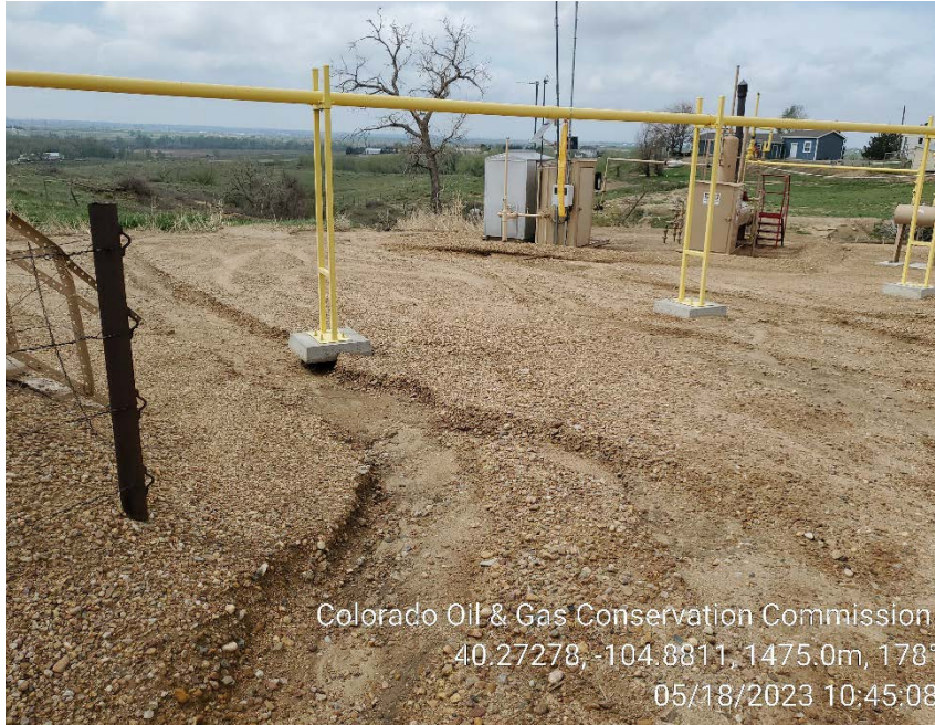
Storm water BMP's on 5/18/2023
