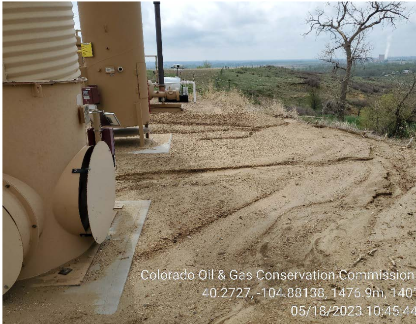
Storm water BMP's on 5/18/2023
