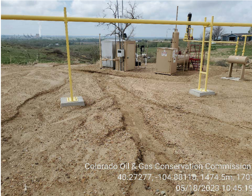
Storm water BMP's on 5/18/2023
