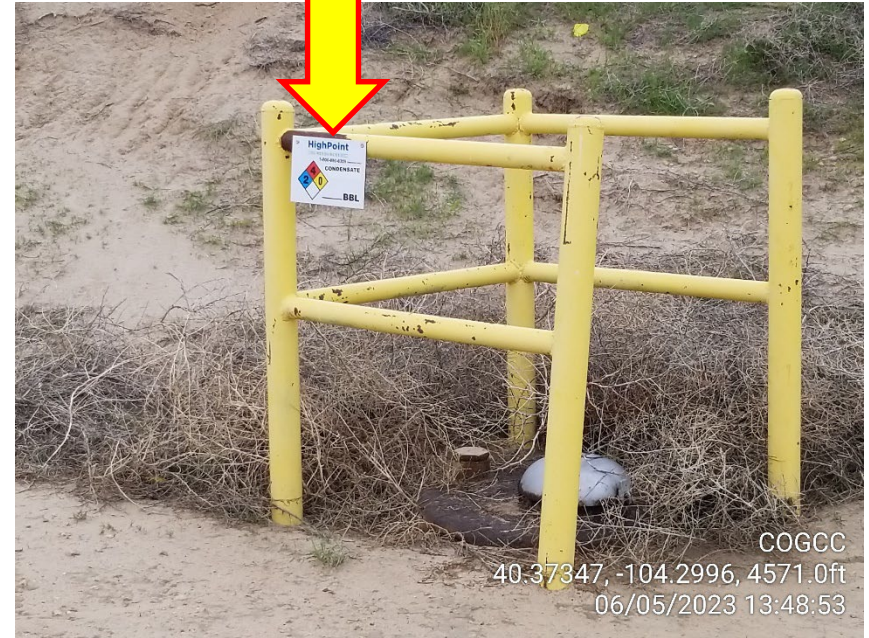
Photo 14 – Missing Capacity Label
