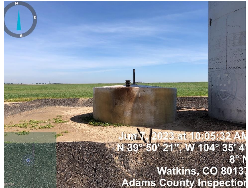
Photo#4 Produced Water Tank/ NO BBL Markings
