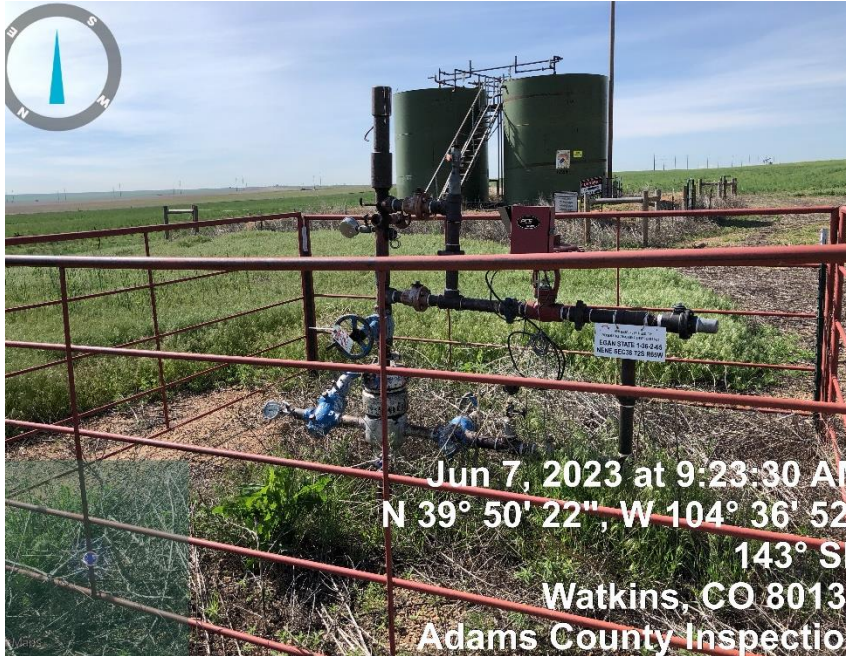
Photo#1 Wellhead/ PACKING Leaking Gas
