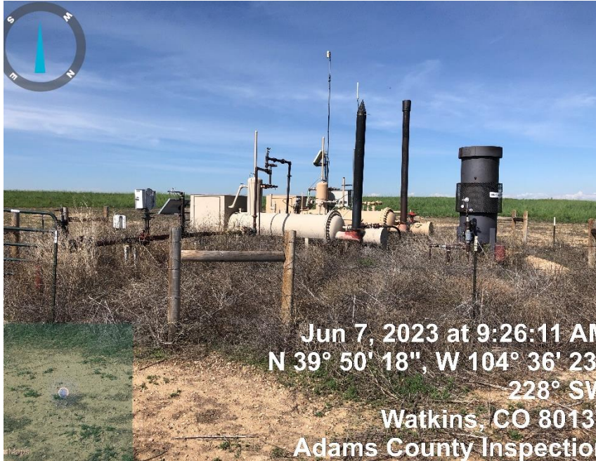
Photo#3 (2) Separators/ECD/Gas Meter
