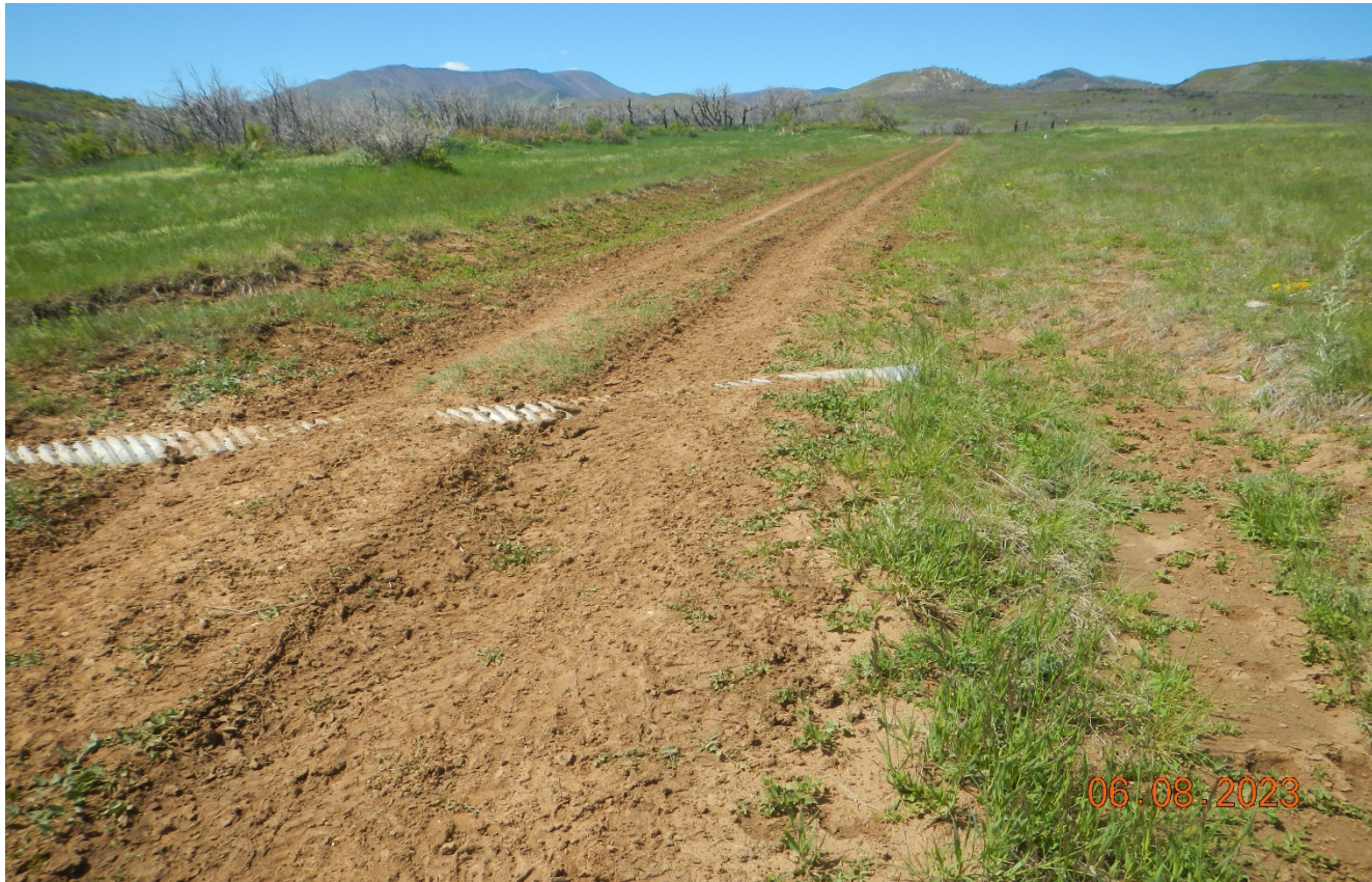
Photo 1. The culvert installed along the access road is not maintained and stormwater is bypassing the culvert. Lat/Long:37.50521,-105.07444. Previous corrective action has not been completed.
