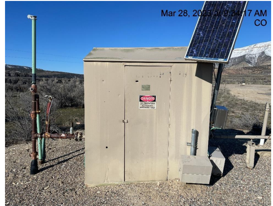
Photo # 3488 From Inspection 708900175 conducted on 03/28/2023 Meter calibration info not conspicuously posted
