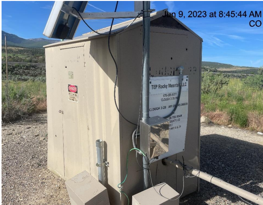
Photo # 9914 Meter calibration info not conspicuously posted
