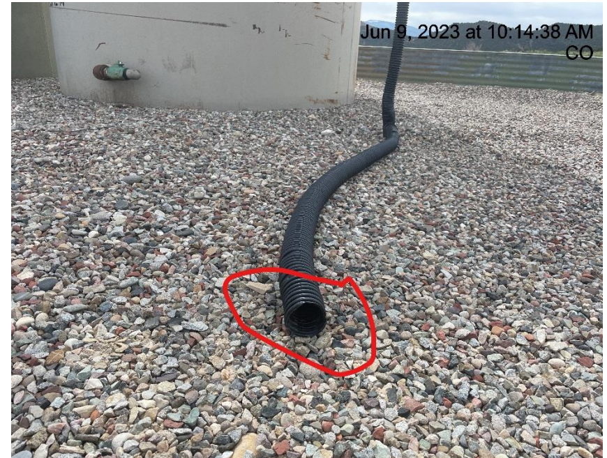
Photo # 9957 Flowline heating insulation open ended
