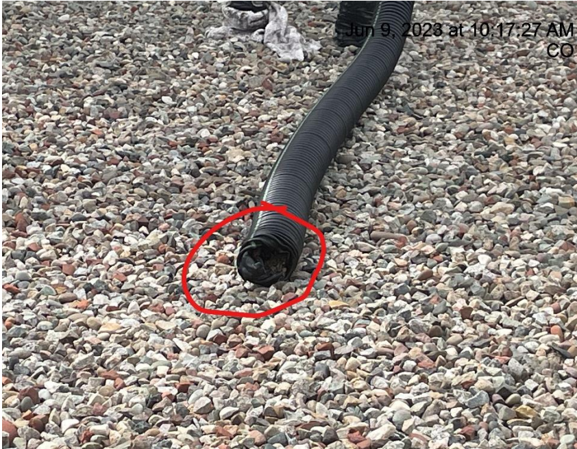
Photo # 9963 Flowline heating insulation open ended
