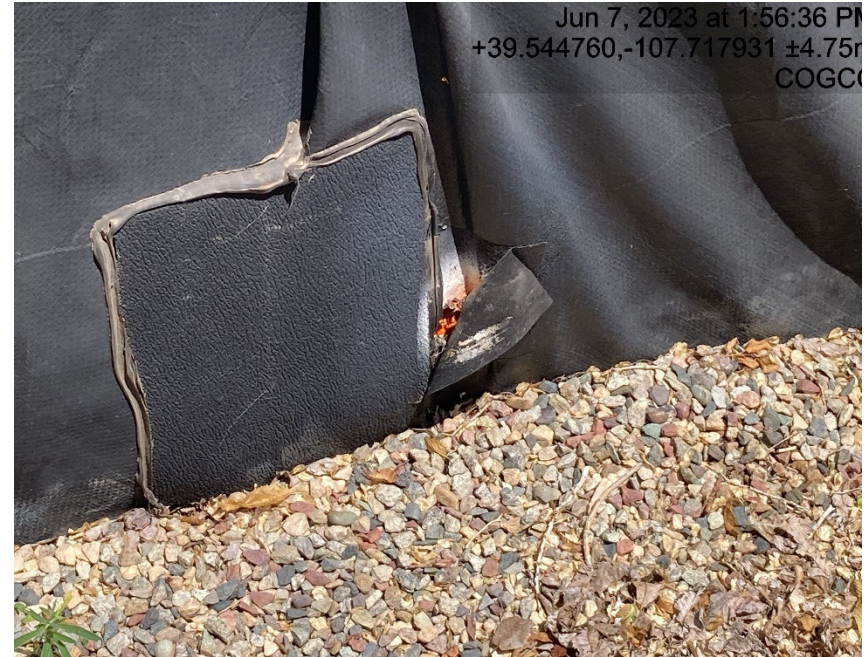
Recent inspection of holes in containment
