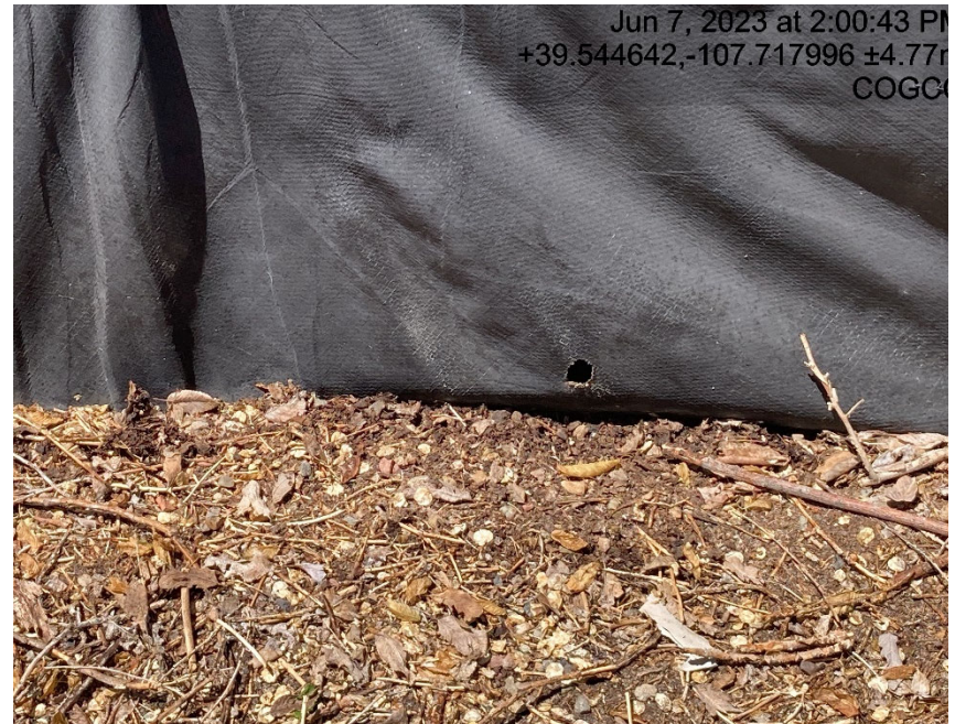
Recent inspection of holes in containment
