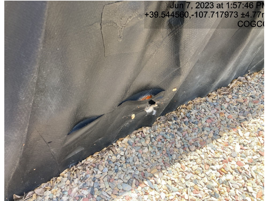
Recent inspection of holes in containment
