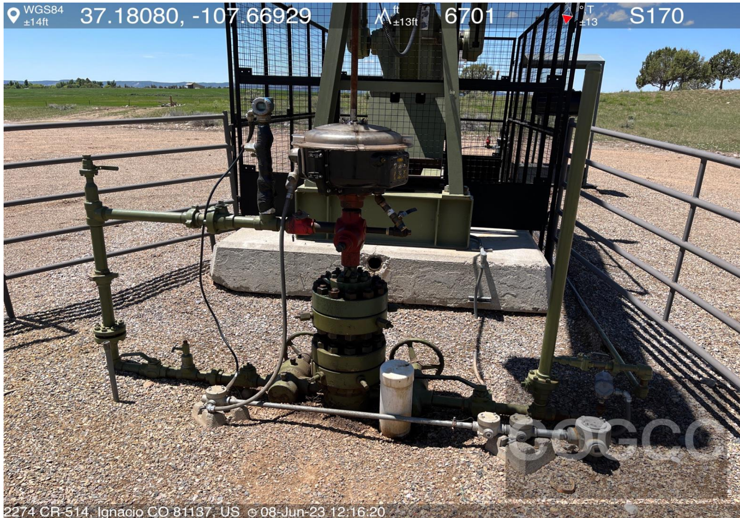
Photo #2. View of wellhead assembly.
