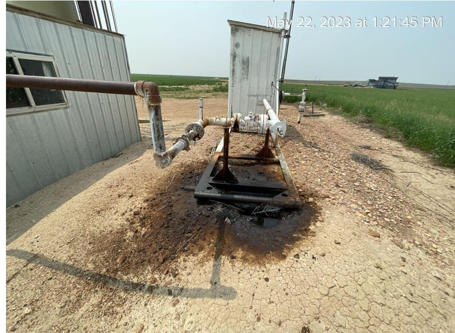
Photo 4. Photo taken of spilled oil from separator on location.
