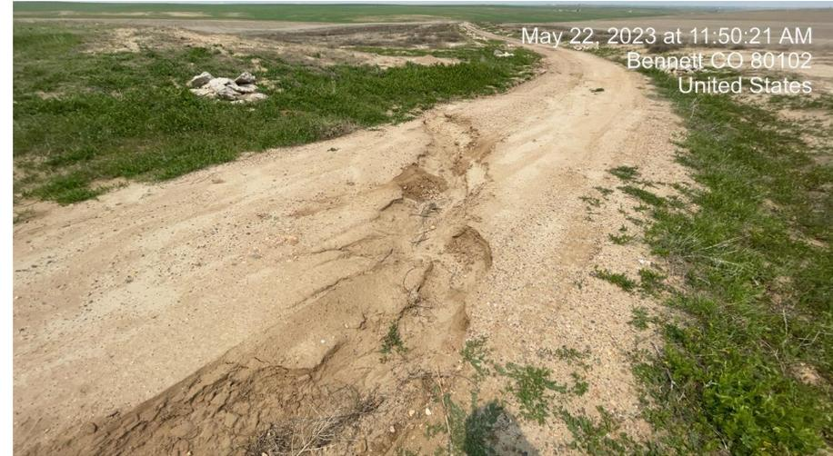
**Photo 3. Photo taken of Weeds, erosion o access road and concrete uses as check dams on site**
