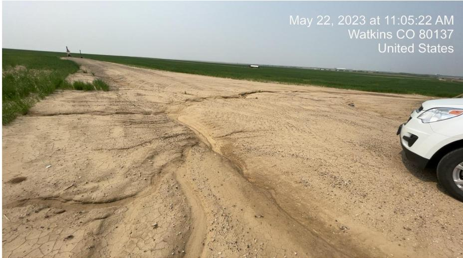
**Photo 3. Photo taken of erosion on site and access road.**
