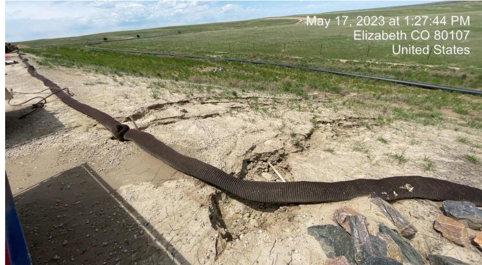
**Photo 11. Photo of pad corner berm collapse.**
