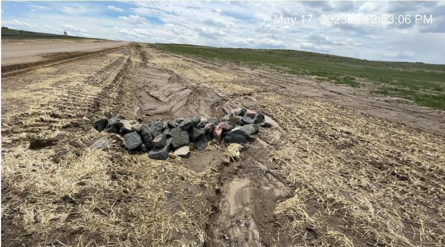
**Photo 3. Photo taken of runoff path going around rock check dams on access rd to site.**
