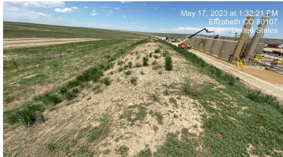
Photo 14. Photo of topsoil stockpile. weeds and bare soil present.
