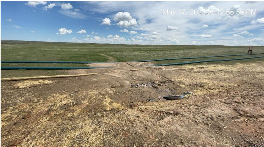
**Photo 7. Photo taken of access road culvert outlet, sediment burning by water lines, and sediment has moved offsite.**
