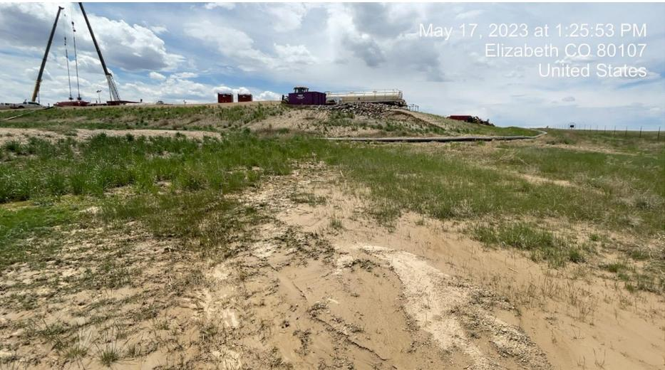
**Photo 8. Photo taken of erosion coming off location due to the corner of the pad collapsing.**
