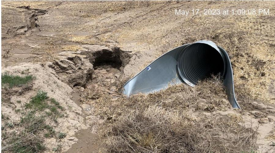
**Photo 5. Photo taken of access road culvert inlet. no rip rap present. erosion and lack of proper soil stabilization.**
