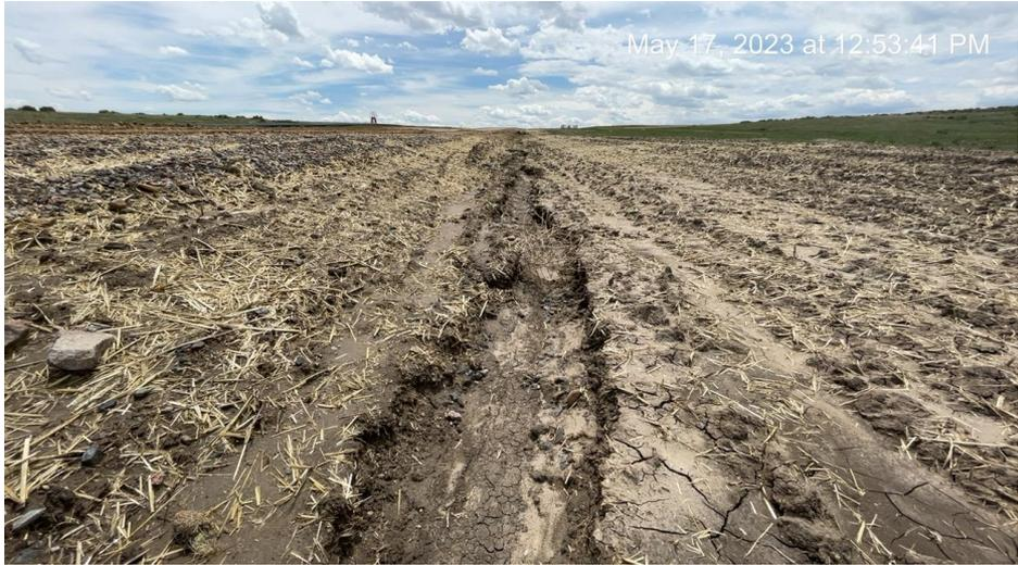
**Photo 4. Photo taken of erosion along access road to site, due to improper soil stabilization.**
