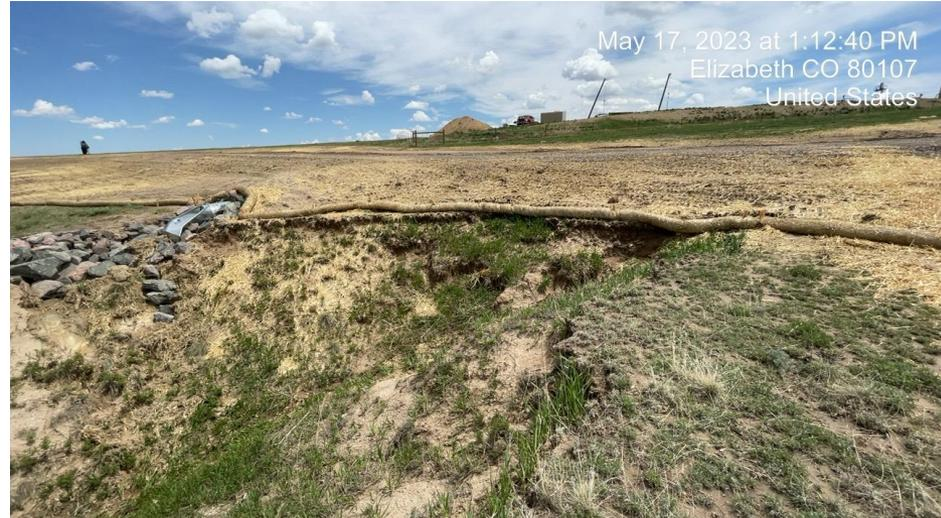
**Photo 6. Photo taken of erosion coming off access road slope, BMP failure, erosion and reeling of roadside.**
