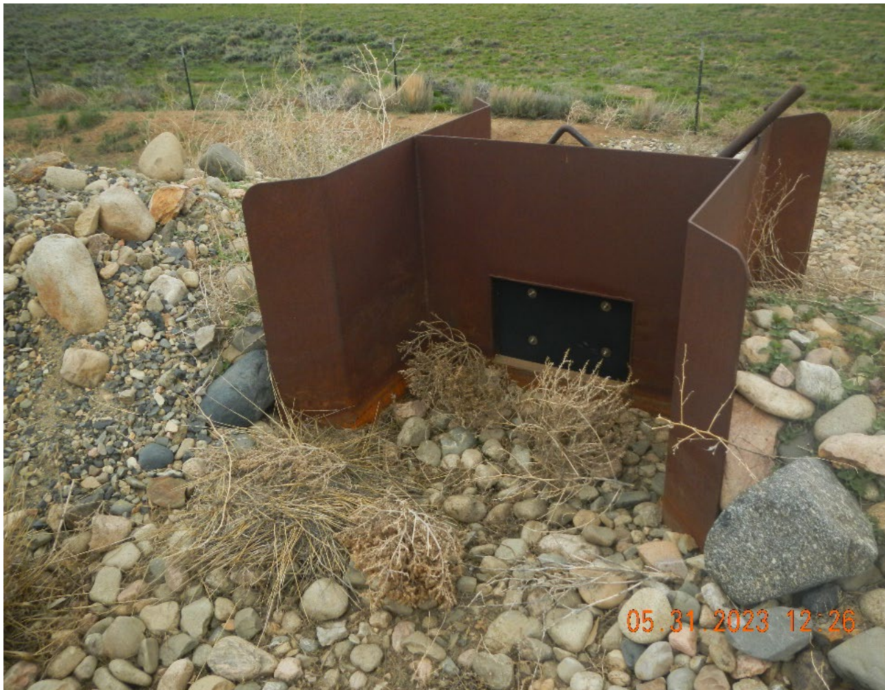
Photo #4 Stormwater gate, in closed position.
