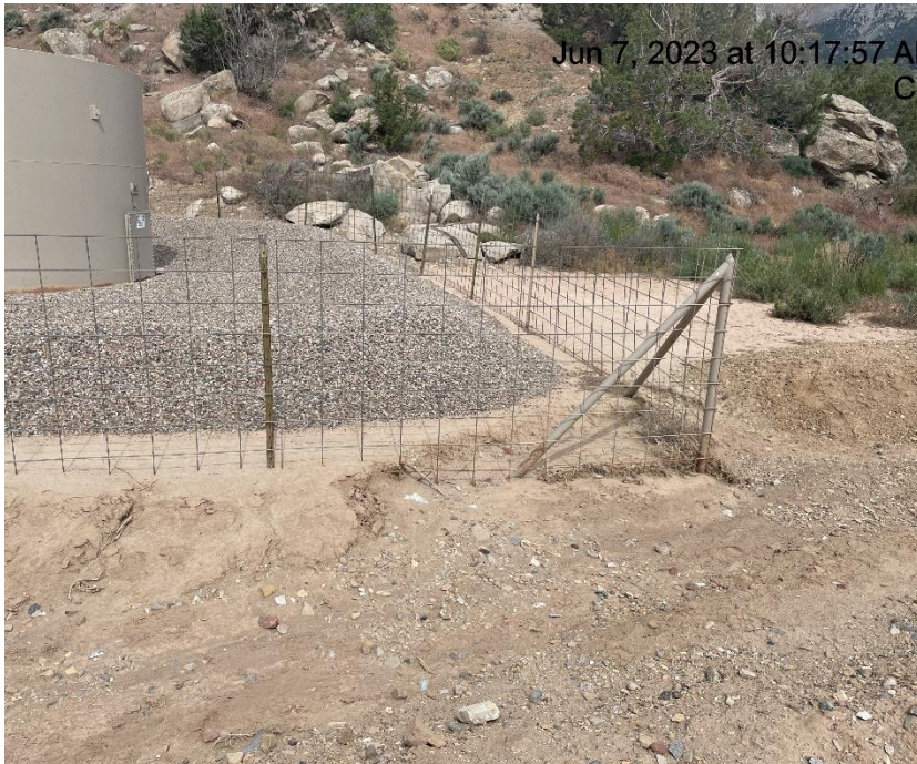
Photo # 9739 Erosion near tank battery containment
