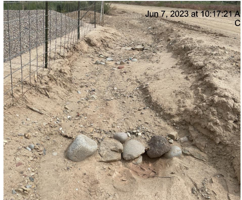
Photo # 9735 Ditch & Check dams need maintenance/erosion near fence & earthen tank battery containment
