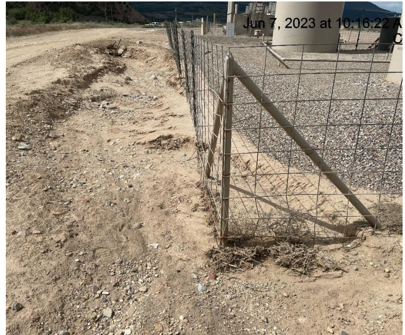
Photo # 9727 Erosion within inches of earthen tank battery containment
