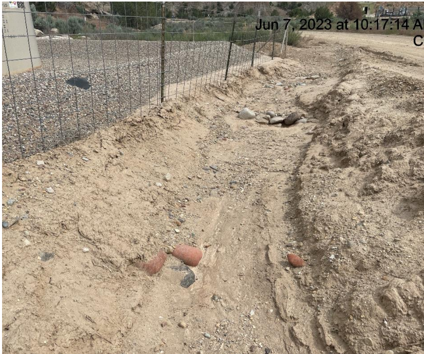
Photo # 9734 Ditch & Check dams need maintenance/erosion near fence & earthen tank battery containment
