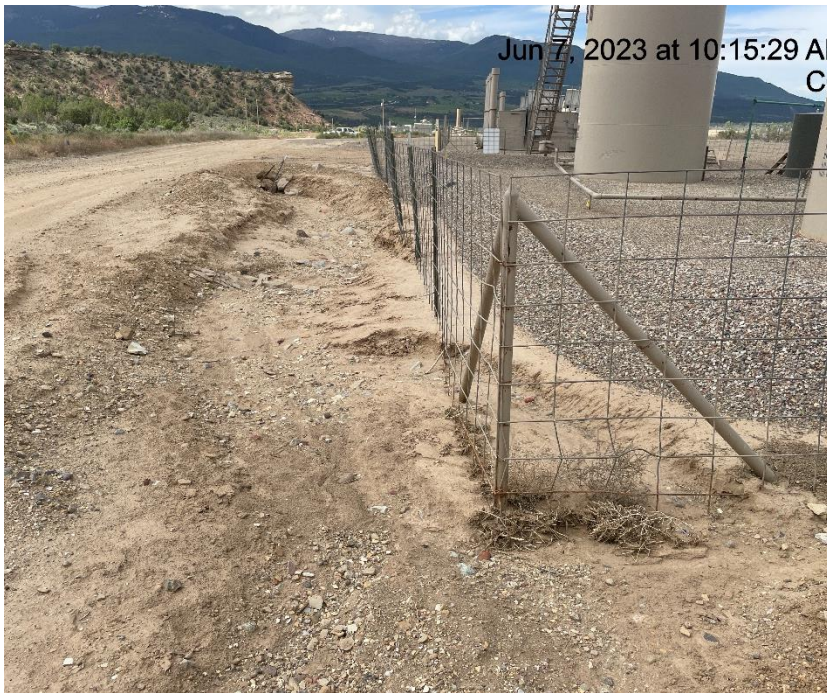
Photo # 9722 Ditch needs maintenance/erosion within inches of earthen tank battery containment
