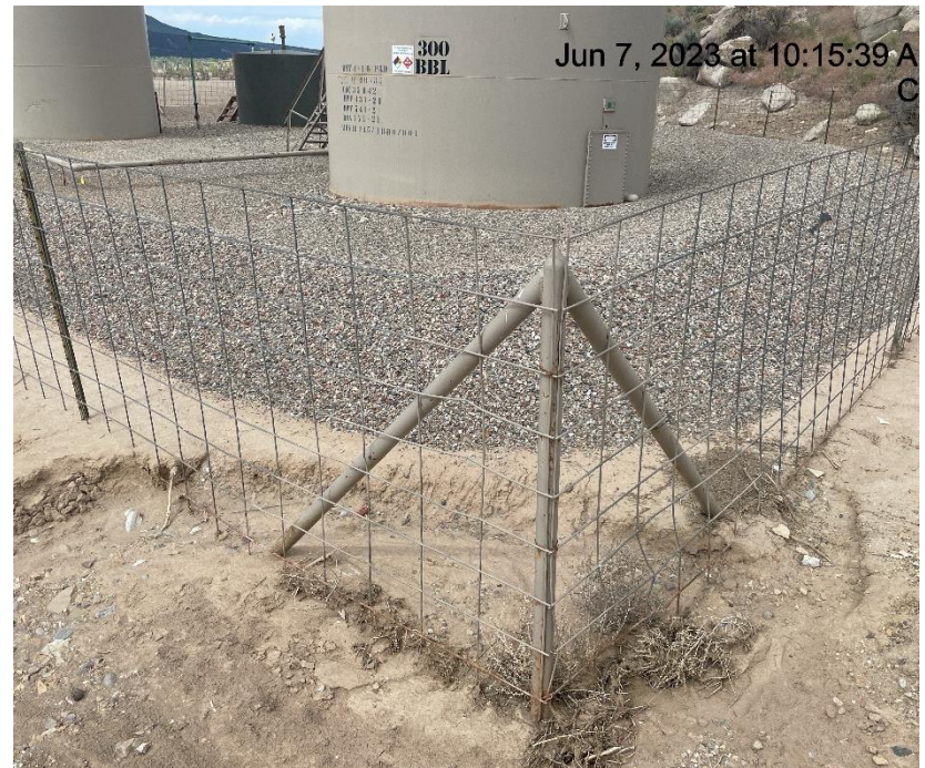
Photo # 9723 Erosion within inches of earthen tank battery containment
