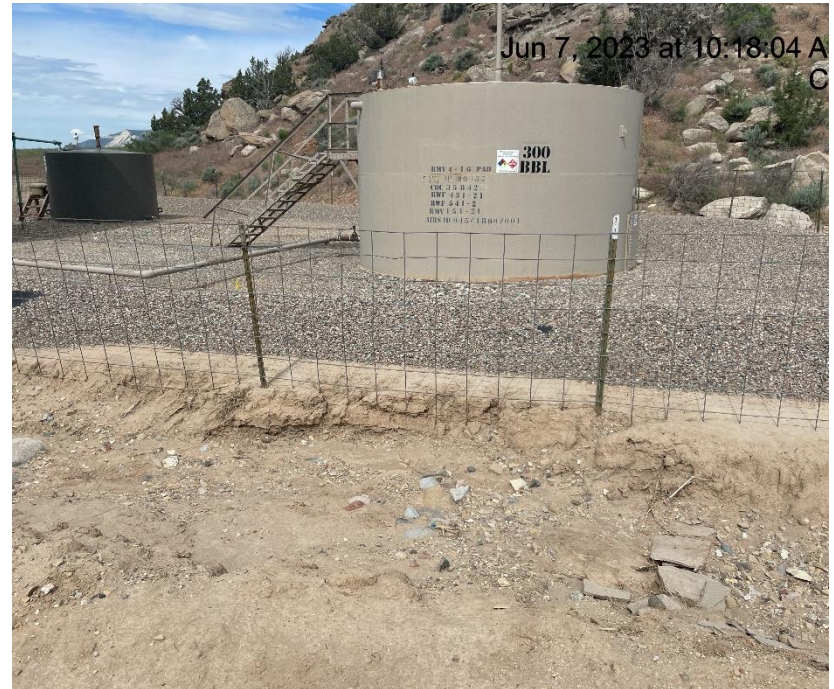
Photo # 9740 Erosion near fence & tank battery containment
