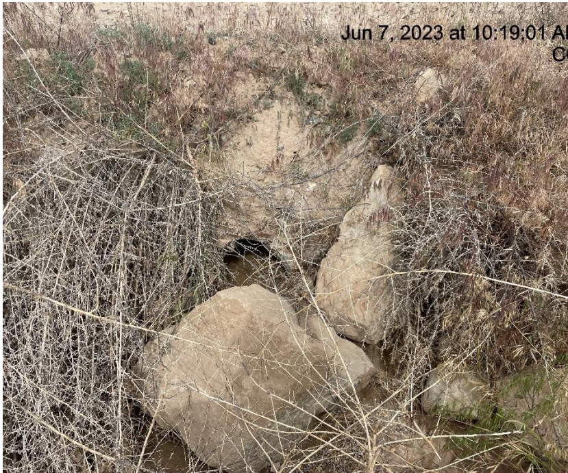
Photo # 9745 Culvert needs maintenance
