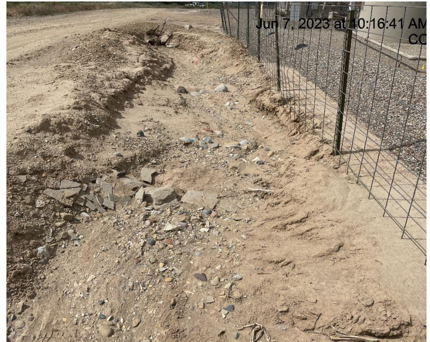
Photo # 9730 Ditch/check dams/culvert needs maintenance
