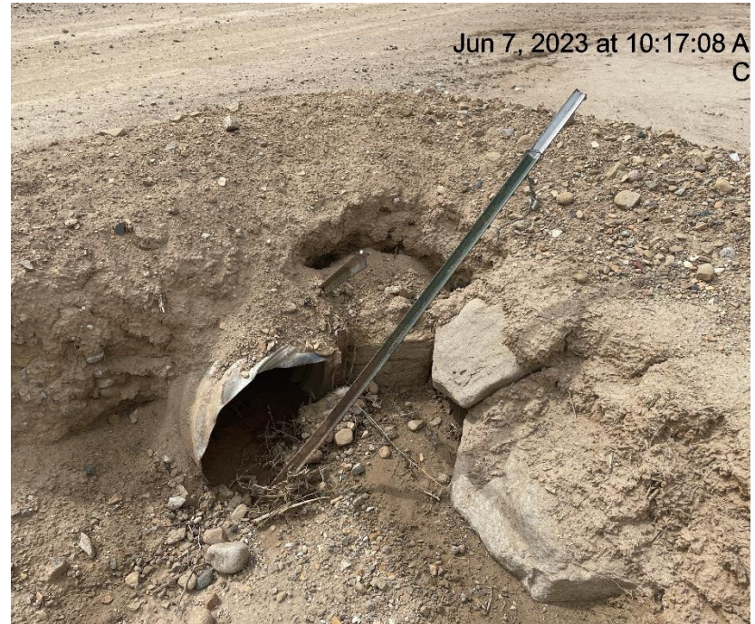
Photo # 9733 Culvert needs maintenance
