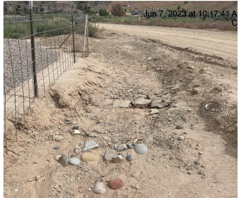
Photo # 9737 Ditch & Check dams need maintenance/erosion near fence & earthen tank battery containment
