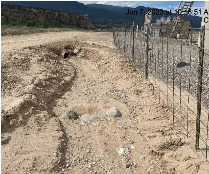
Photo # 9731 Ditch/check dams/culvert needs maintenance
