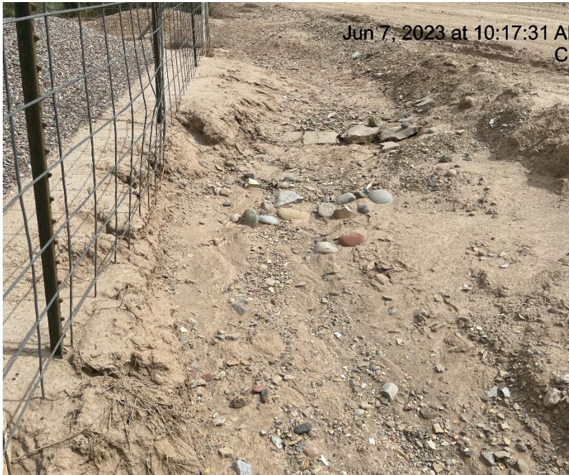
Photo # 9736 Ditch & Check dams need maintenance/erosion near fence & earthen tank battery containment
