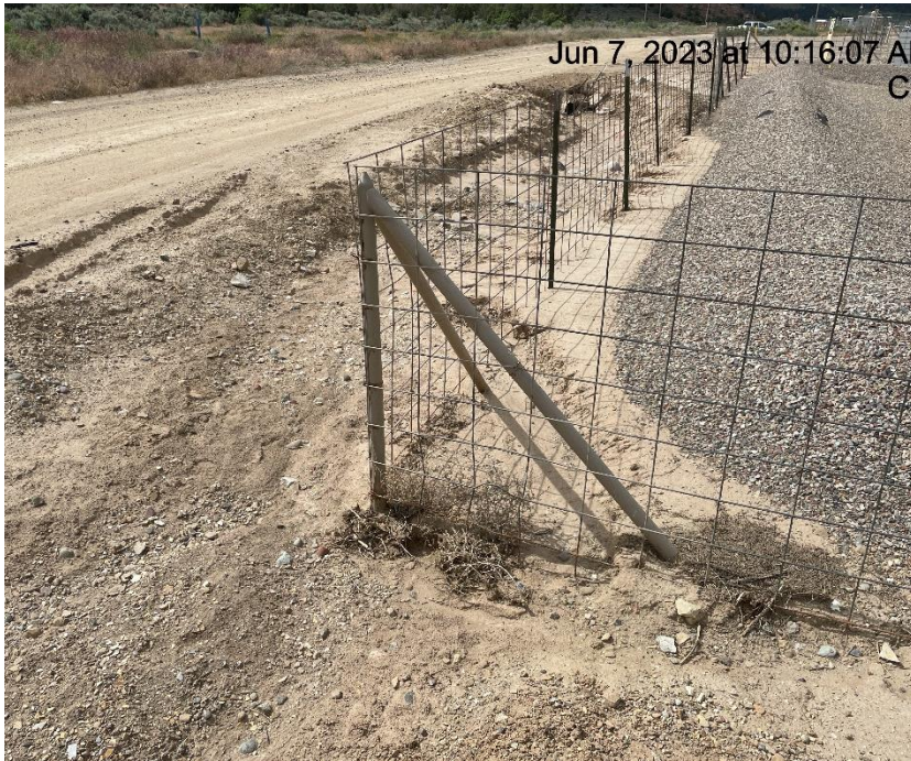
Photo # 9725 Erosion within inches of earthen tank battery containment
