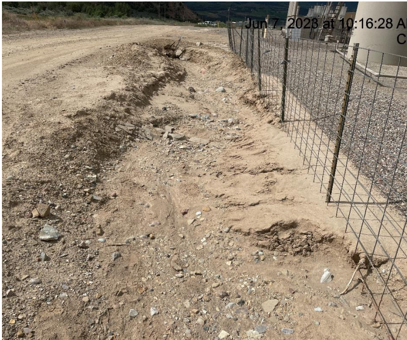
Photo # 9728 Ditch/check dams/culvert needs maintenance
