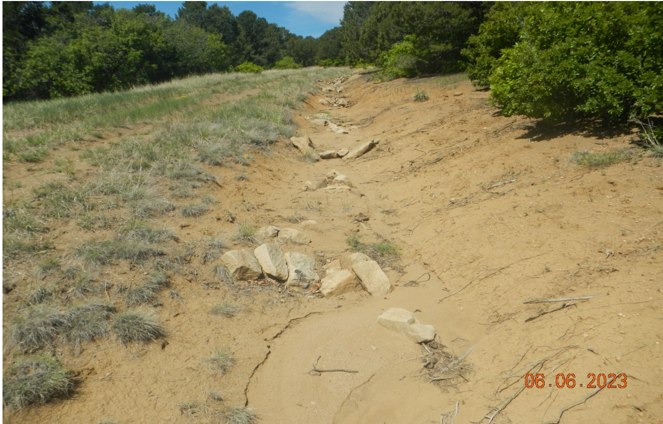
Photo 1. Facing southwest along the former access road. The road was not recontoured and reclaimed. There is erosion occurring along the road and the rock check dams are displaced. Previous corrective action was not performed.
