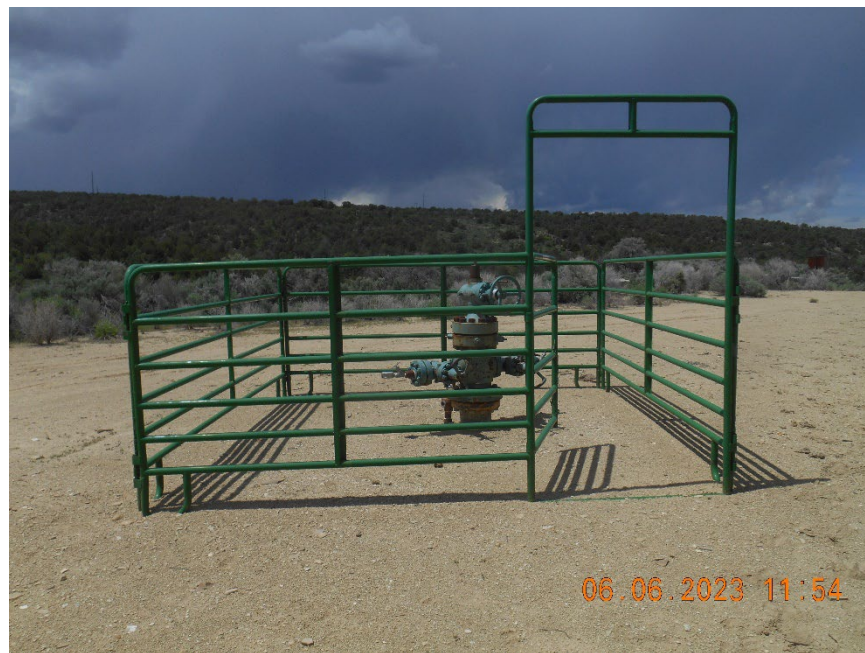
Injection wellhead with fence. Temporarily Abandoned
