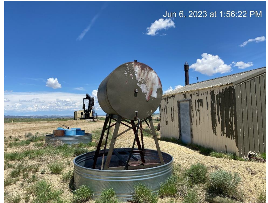
Unidentified tank missing required labels
