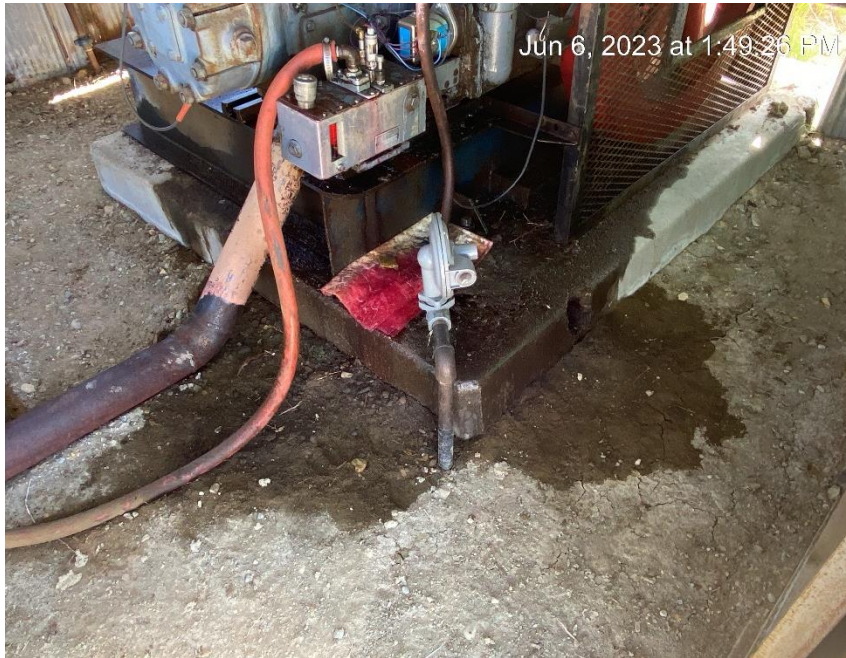
Oil leak. Stained equipment and soil
