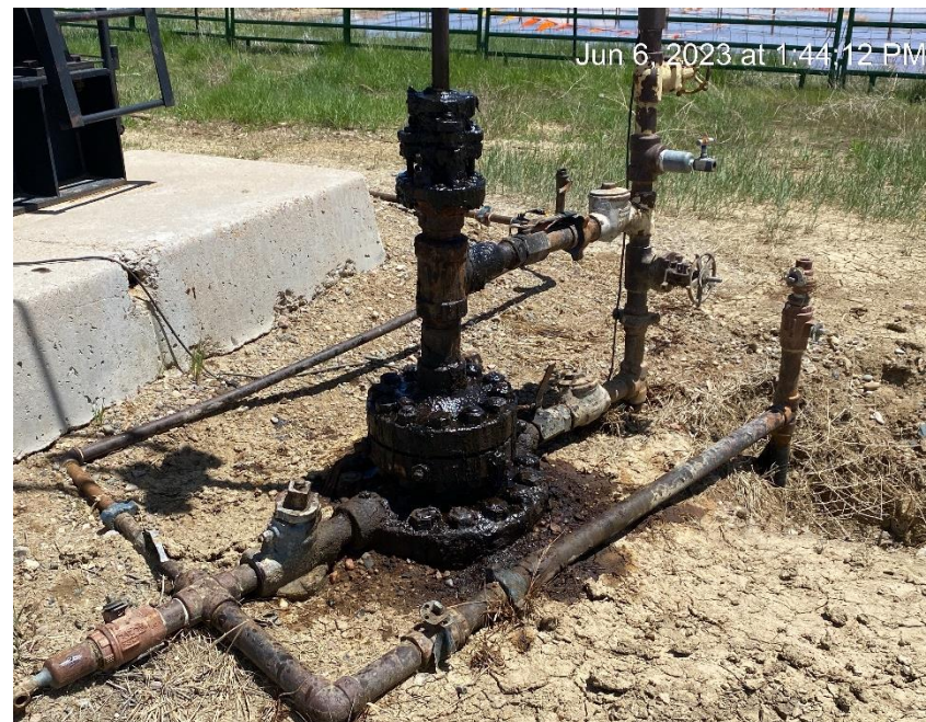
Leaking equipment. Stained equipment and soils
