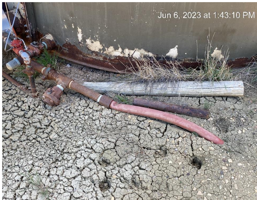
Open end tank valve. Debris
