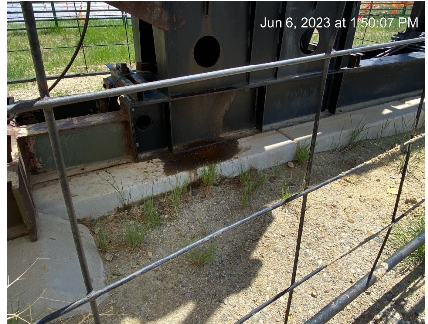
Oil leak. Stained equipment and soil
