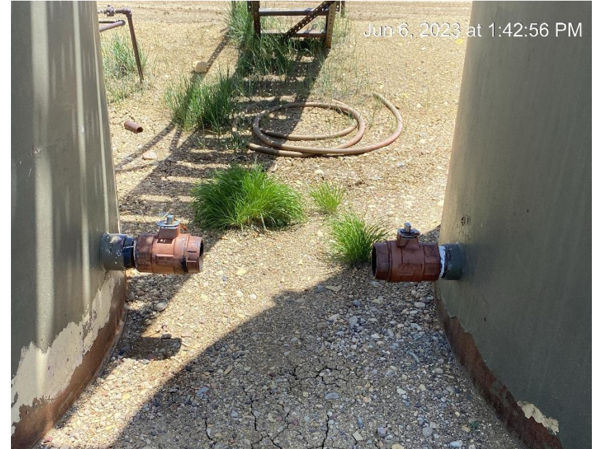
Open end tank valves. Debris
